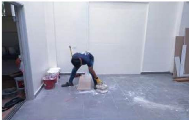
Photo 3.18 Cleaning up after Installation
