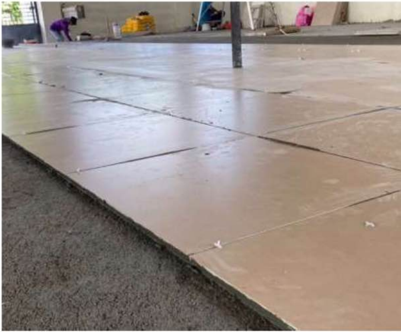
Photo 3.14 Spacers between the tiles for same spacing and levelling
