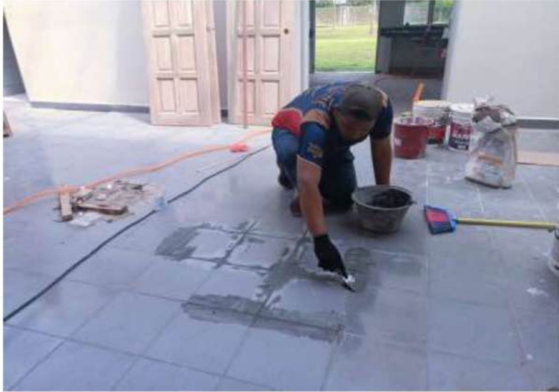
Photo 3.17 Spreading the grout joints process
