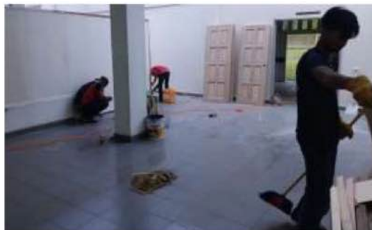
Photo 3.19 Cleaning up after Installation
