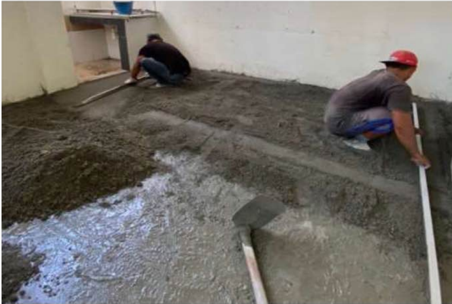
Photo 3.4 Mortar spot pegging are prepared to provide correct levels
