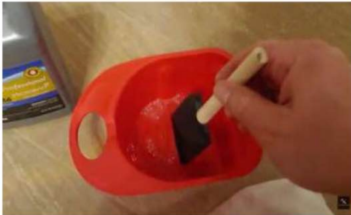
Photo 3.42 Sealing the grout
