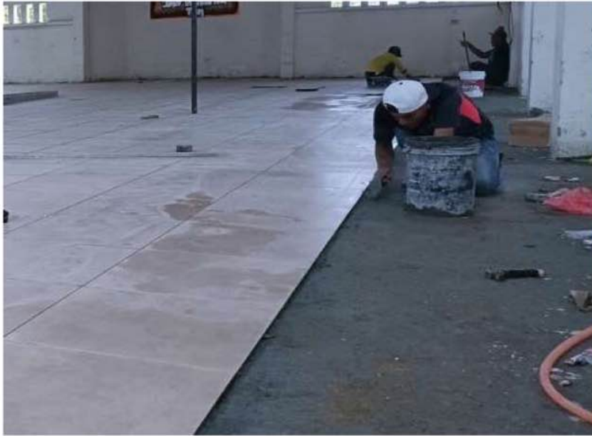
Photo 3.12 Apply and laying the SikaCeram-88 adhesive type
