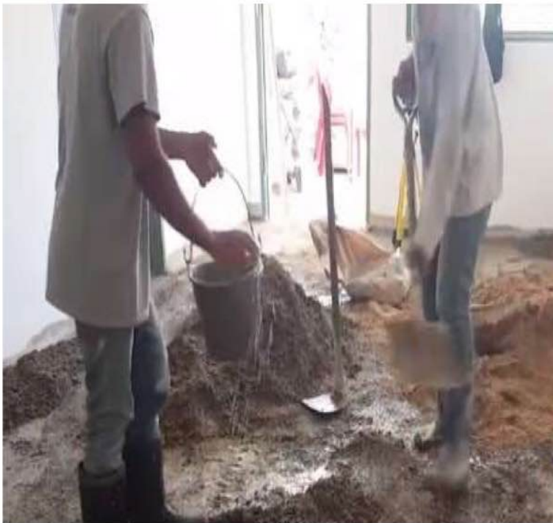
Photo 3.2 Prepare the cement render with the right ratio
