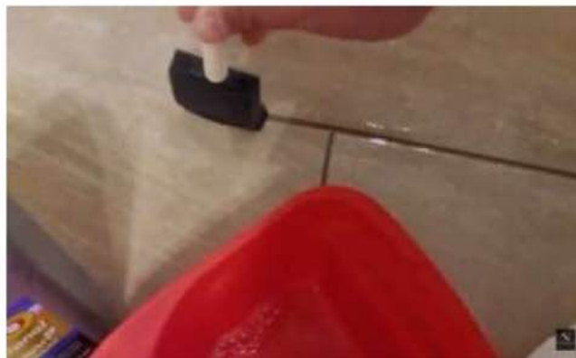
Photo 3.43 Sealing the grout
