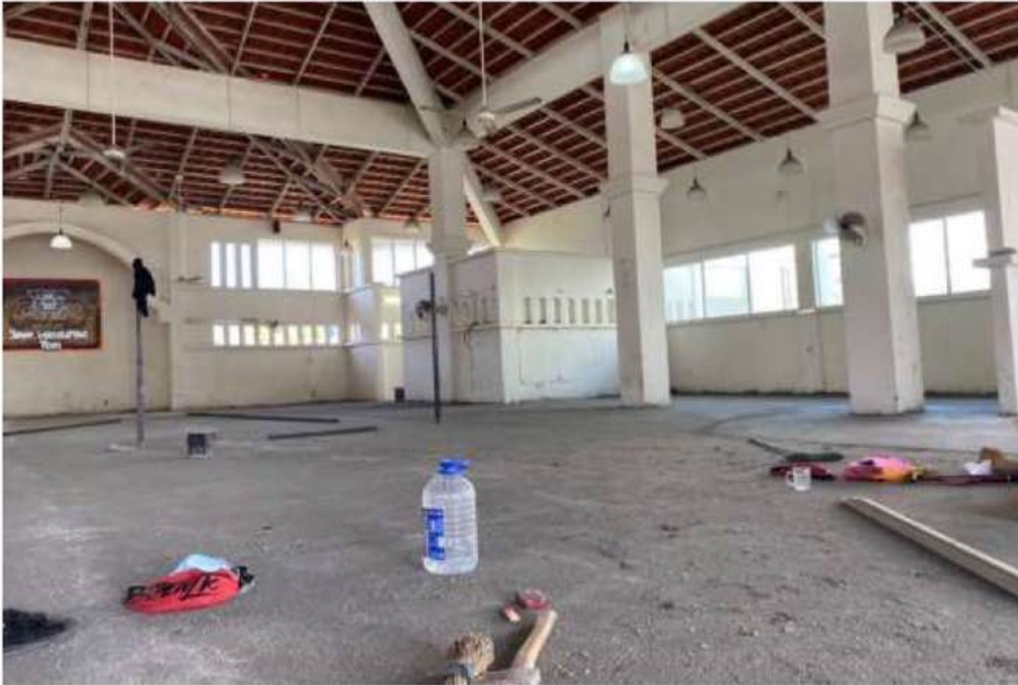
Photo 3.8 Finished the Cement Render
