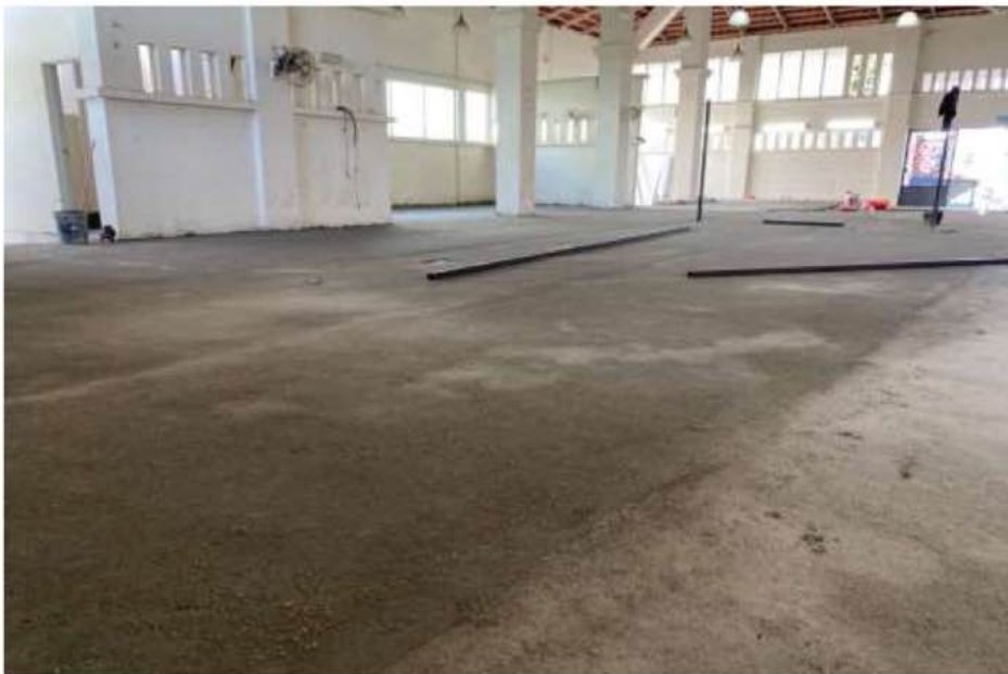
Photo 3.9 Finished the Cement Render before Installation tiles
