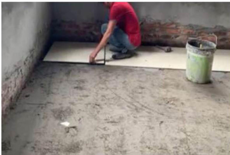
Photo 3.13 Set tile for installation
