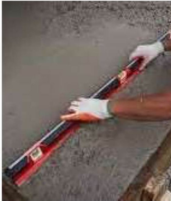
Photo 3.28 Spirit Level in order to check the Surfaces are Level
