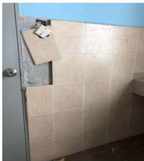
Photo 2.11 Repair of the Wall tiles and Electrical
