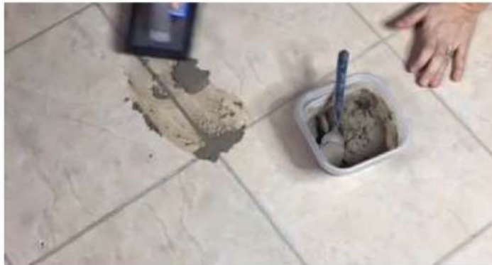
Photo 3.44 Restoration of grout
