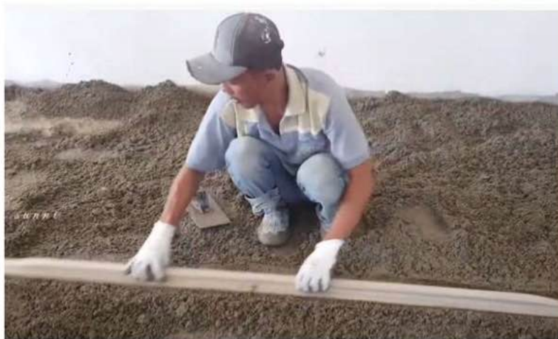
Photo 3.5 Mortar spot pegging are prepared to provide correct levels
