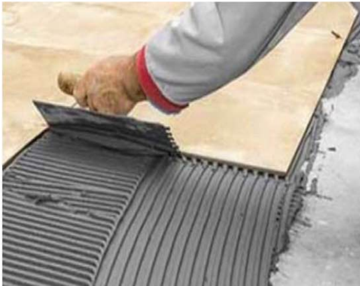
Photo 3.11 Lay mortar and Adhesive
