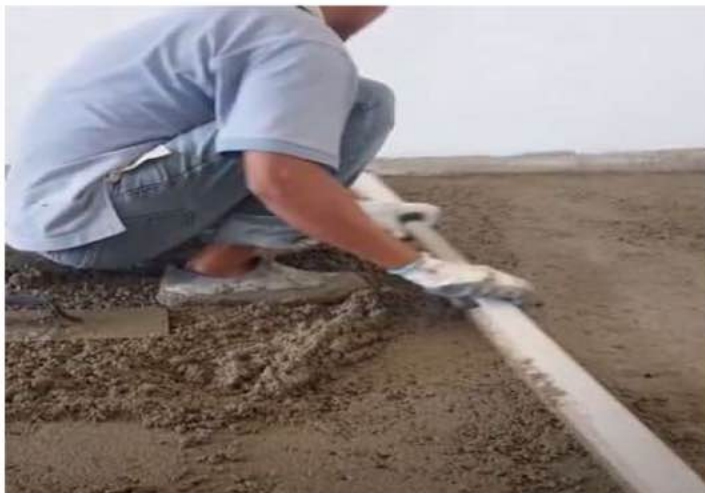
Photo 3.7 Further level the surface condition
