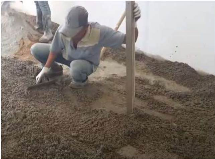
Photo 3.6 Laid Cement Render which are the Mixture of that four Material Combine
