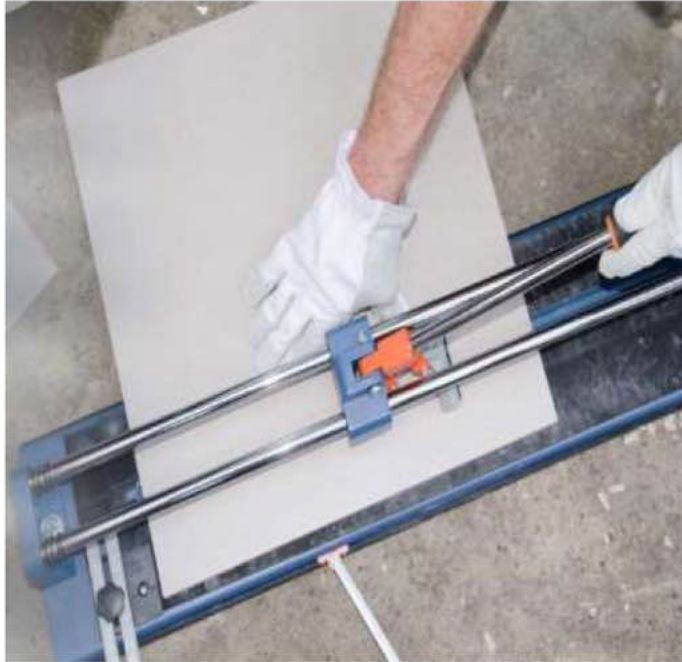
Photo 3.21 Cutting tiles manually using Tile Cutter
