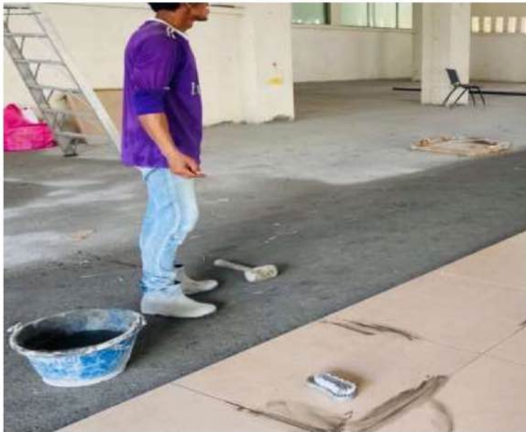
Photo 3.16 Spreading the grout joints process
