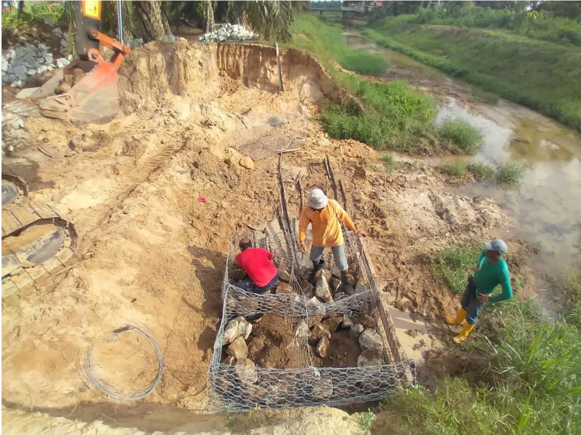
Figure 2.4.5 Gabion wall construction.
