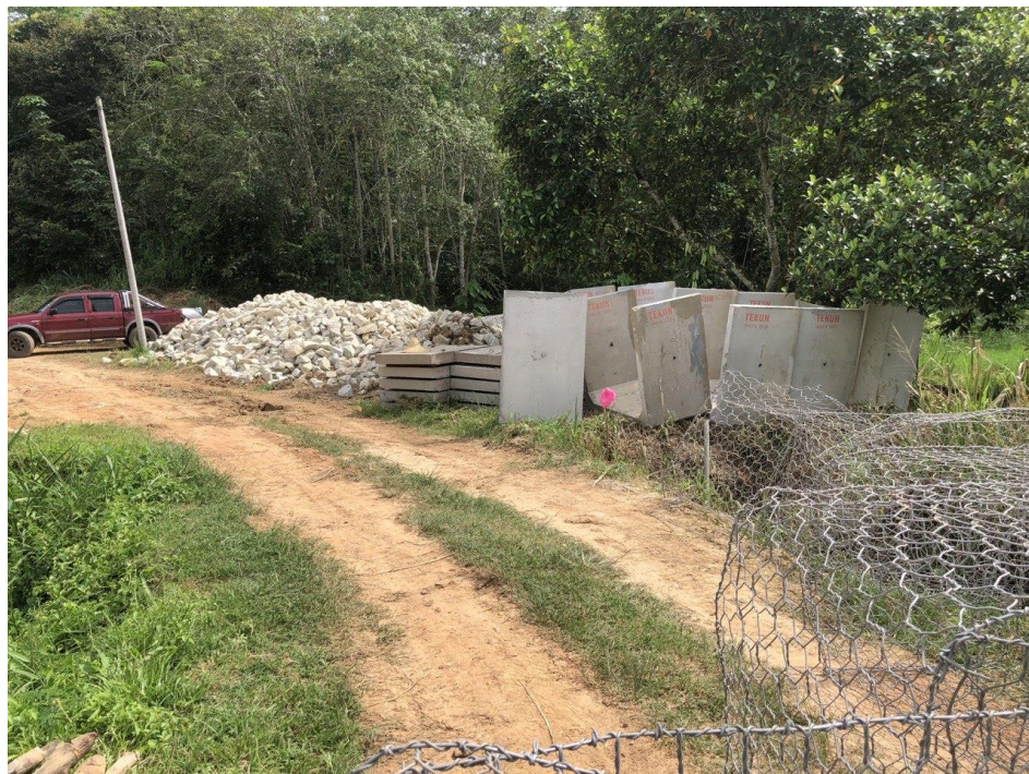
Figure 3.1 The material for gabion wall construction.
