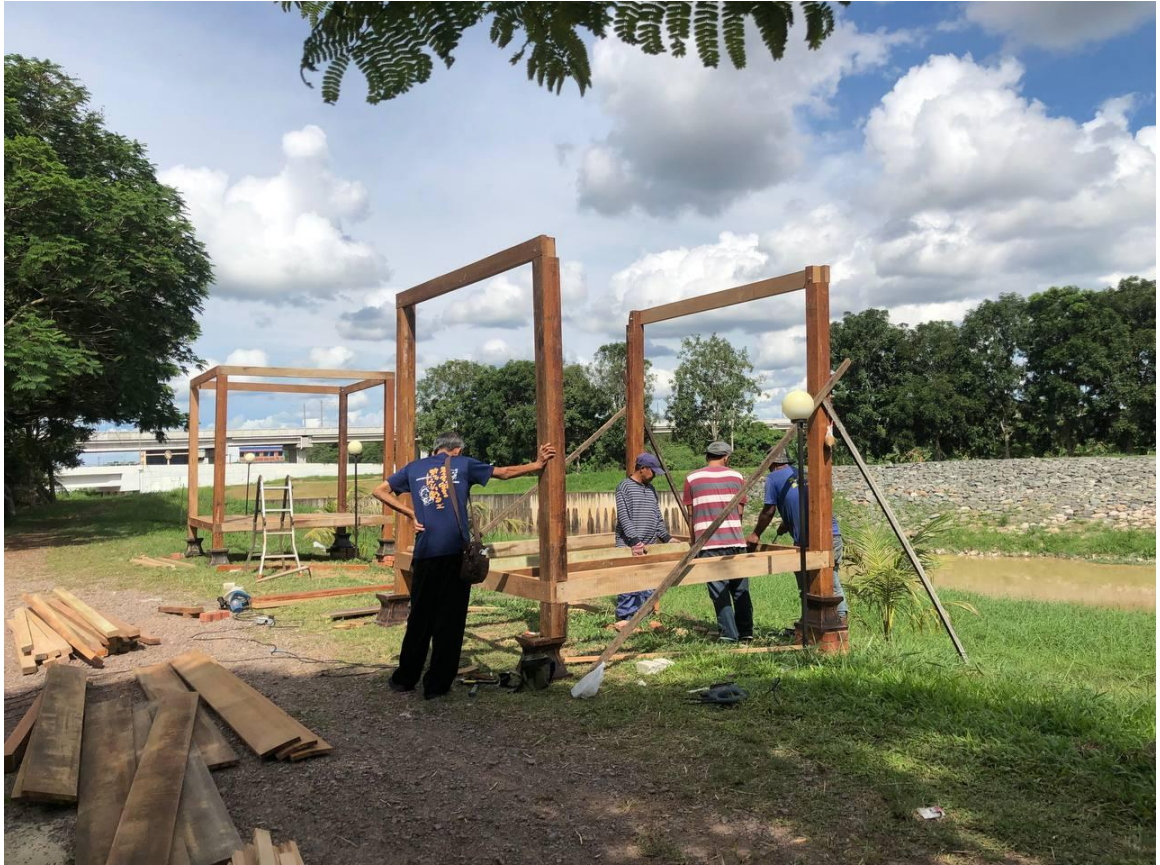
Figure 2.4.1 installing gazebo.
