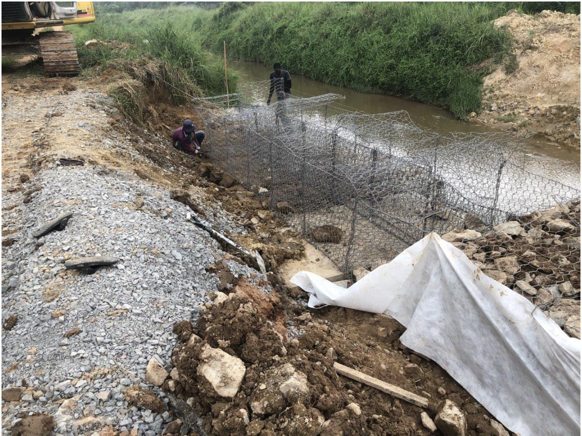
Figure 2.4.7 Gabion construction.
