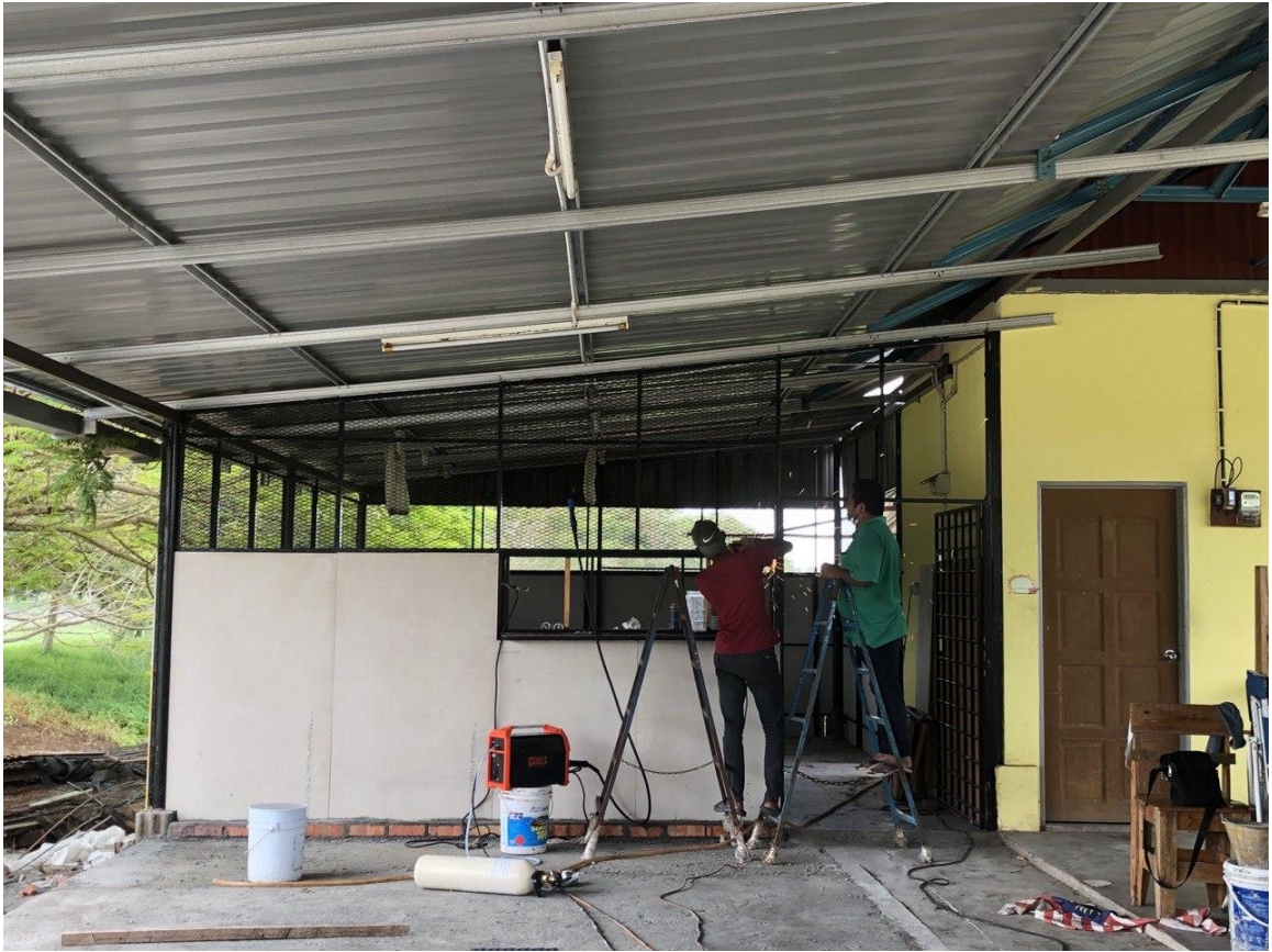
Figure 2.4.9 installing partition as kitchen wall.
