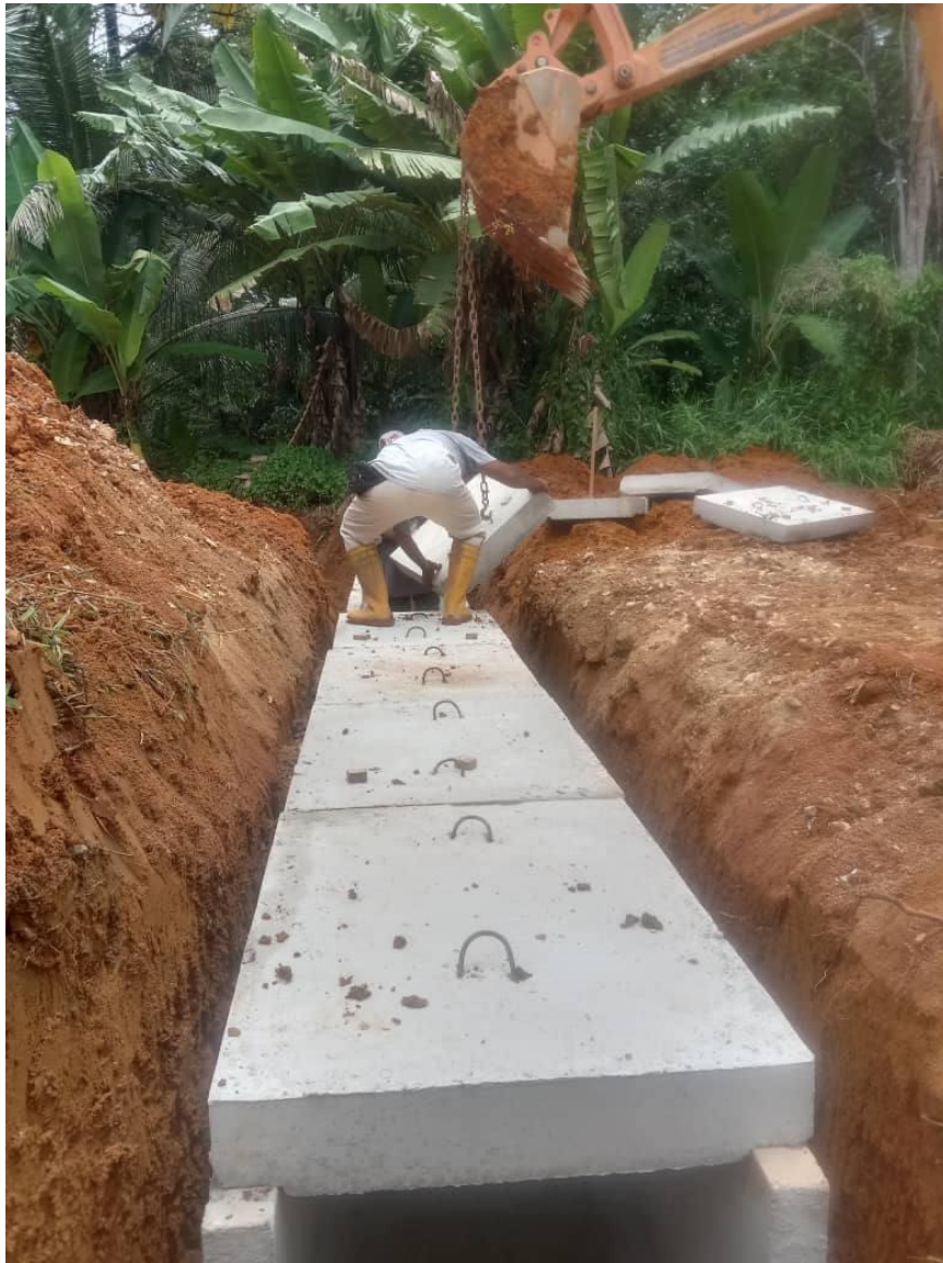
Figure 2.4.2 Installation of culvert.
