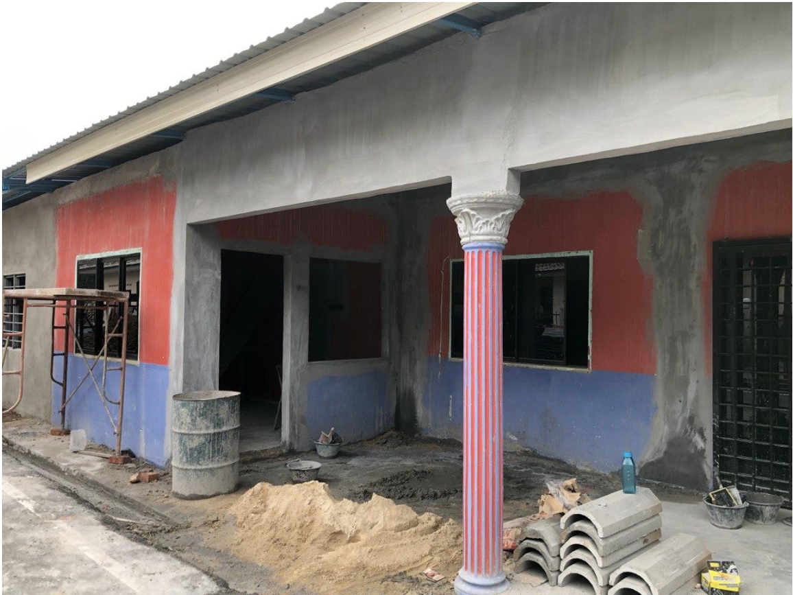
Figure 2.4.8 Renovation of Balai Raya Kg Lubok Kepong .
