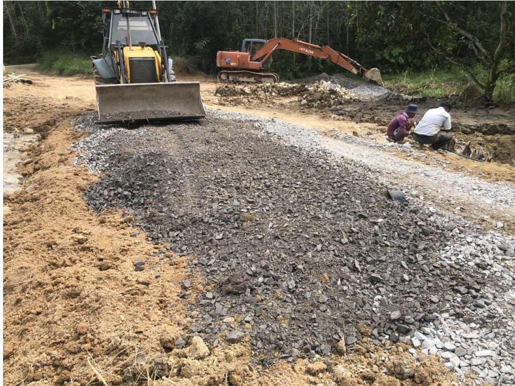
Figure 3.4 put crusher run on top of the road.
