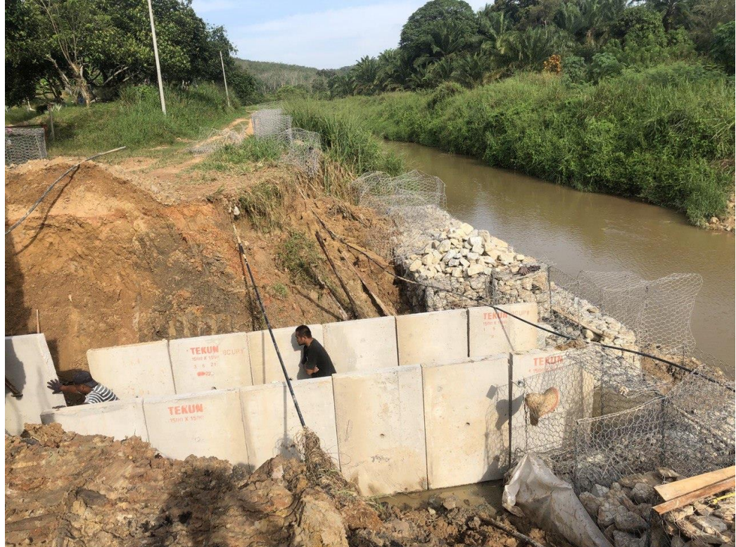
Figure 3.3 Installing culvert.
