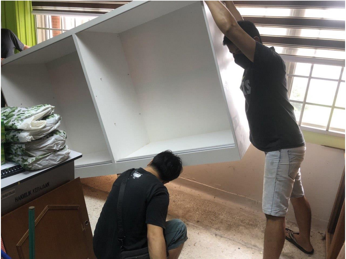
Figure 2.4.10 installing the cabinet.
