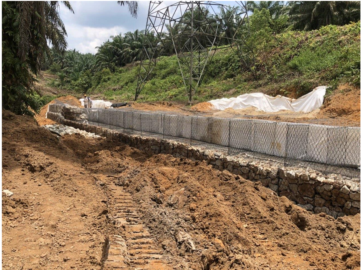
Figure 2.4.3 Gabion wall construction.
