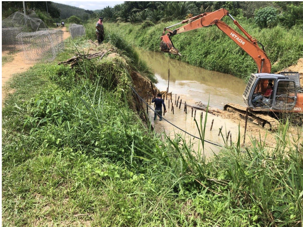
Figure 3.2 Plant the mangroves tree trunks.
