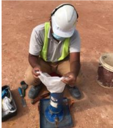
Figure 3.19 pouring sand into cone
