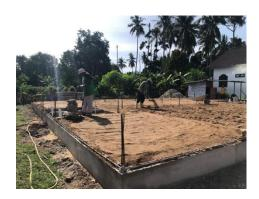
Figure 22: fill the space with the sand and use compactor machine
