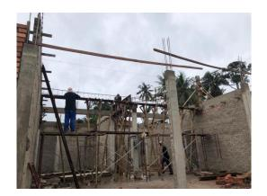
Figure 28: Install reinforment for the beam
