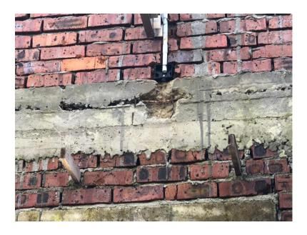
Figure 38 Steel bar visible out from structure
