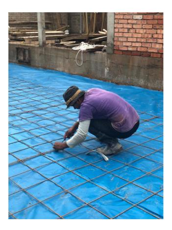
Figure 7 Fixing the BRC
