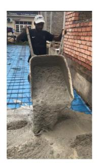
Figure 11 Concretor is pouring the fresh concrete
