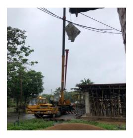
Figure 34 : Concrete pouring using crane and readymix concrete
