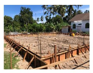
Figure 19: placement of reinforcement and formwork installation
