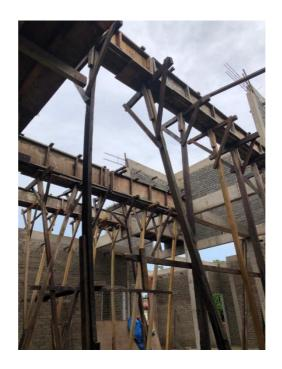
Photos 15 Installation of formwork for roof beam
