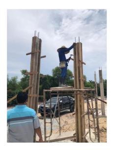
Figure 12 Stripping of formwork
