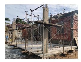
Figure 32: Staging scaffolding installment
