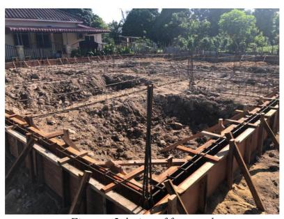
Figure: 5 design of formwork
