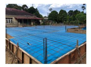
Figure 24: Put plastic sheet under the reinforcement that tie by the wires
