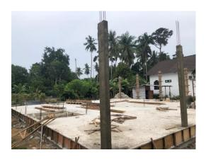
Figure 26: Concrete column construction process
