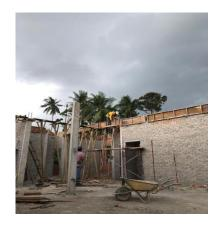
Figure 27 : Preparing Beam formwork
