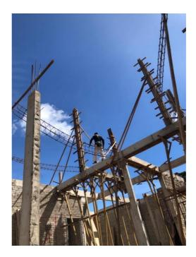
Figure 13 Formwork of beam
