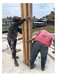
Figure 10 Inspection the vertically before concreting
