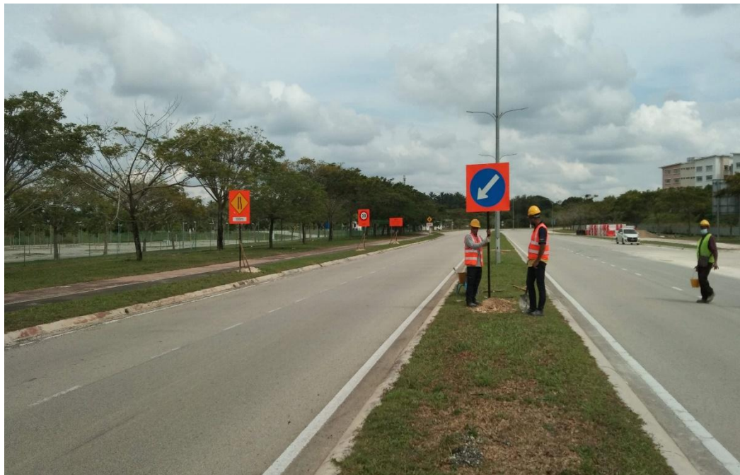
3.21 Install Temporary Signage
