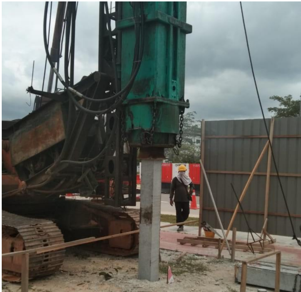
Figure 3.3 Piling Work
