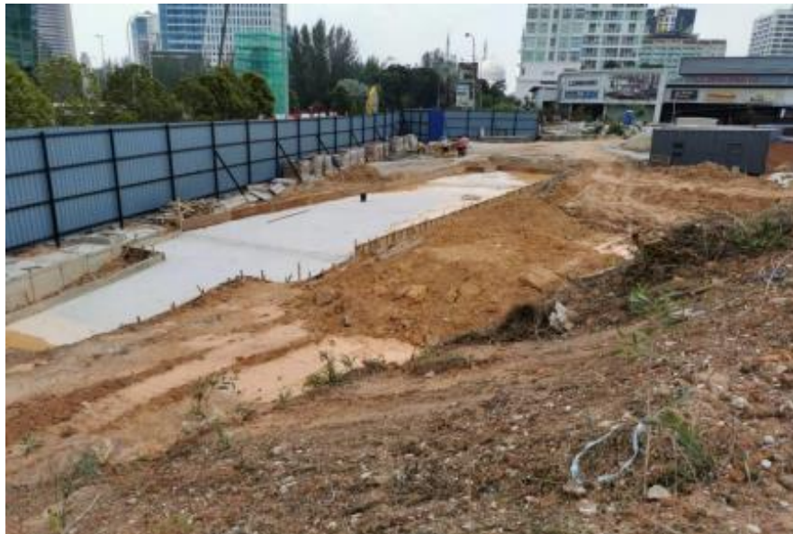
Figure 2.0: Front view (right side) of the project at 20% progress.
