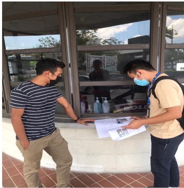
Photo 3.7: The architect of Dekad Wangsa Sdn Bhd (right) attending a site visit with main contractor (left)
