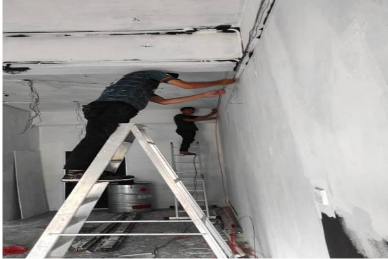
Photo 3.3: Wiring work at Subang Jaya, Selangor
