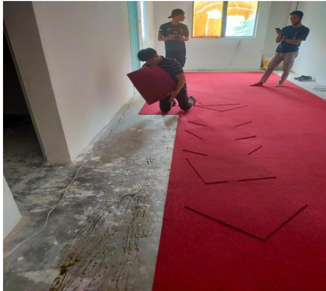
Photo 3.10: The installation of carpet tiles
