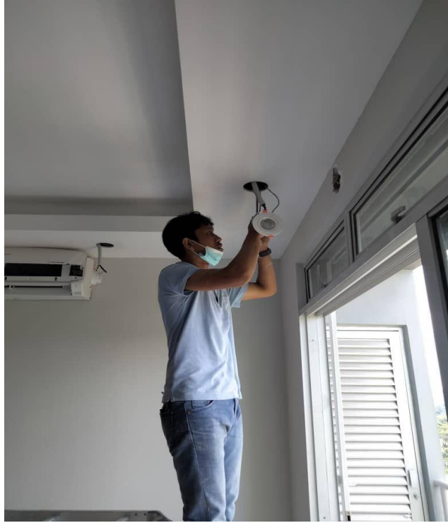
Photo 3.20: Aesthetic lighting installation in the living room
