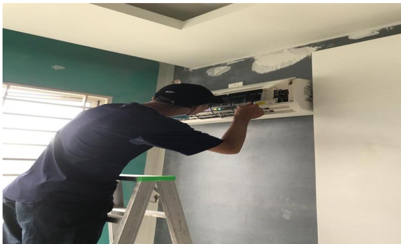
Photo 3.5: Maintenance work on air-conditioner
