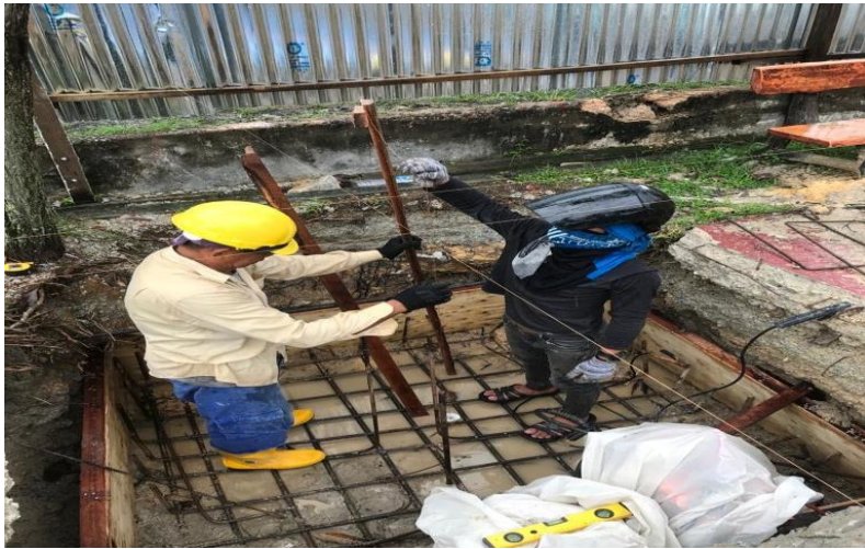
Photo 3.4: Construction of foundation for roof structure at futsal court
