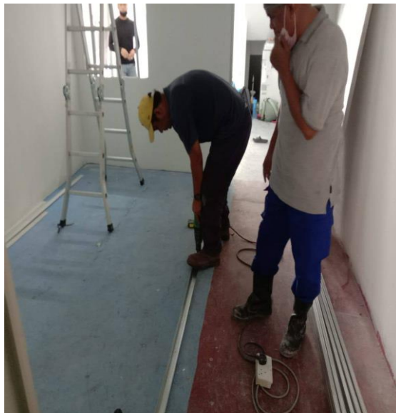
Photo3.13: The installation of partition board at Subang Jaya
