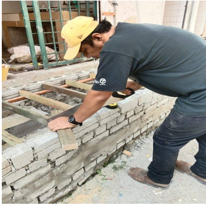
Photo 3.16: The installation of reinforced concrete slab
