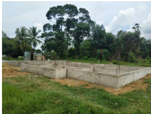
Figure 3.10: Plinth Beam or Slab
