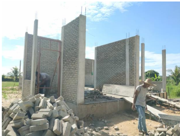
Figure 3.12: Brick Masonry Work
