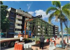
Figure 3.5: Lift up the frame structure using the crane to put on the slab
