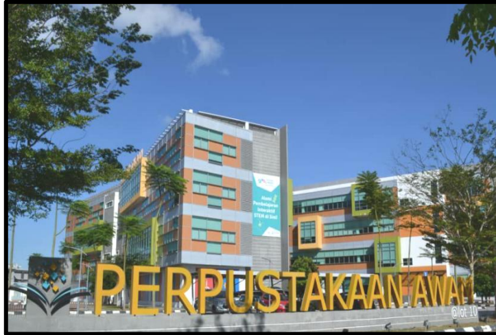
Figure 3: Main building Perbadanan Perpustakaan Awam Pahang (PPAP)
