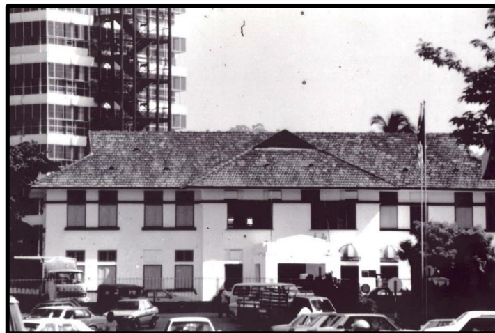
Figure 2: Old Library Building Perbadanan Perpustakaan Awam Pahang (PPAP)
