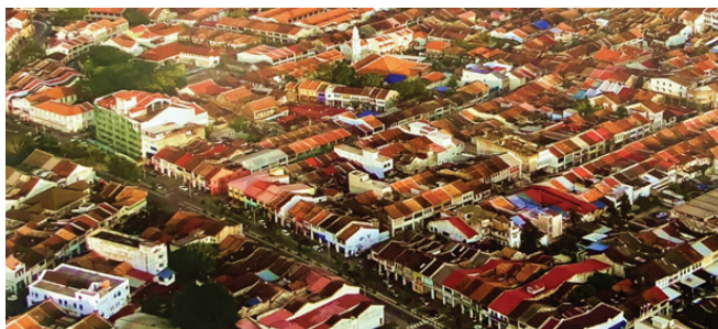
Figure 1. George Town Historic District Aerial View
