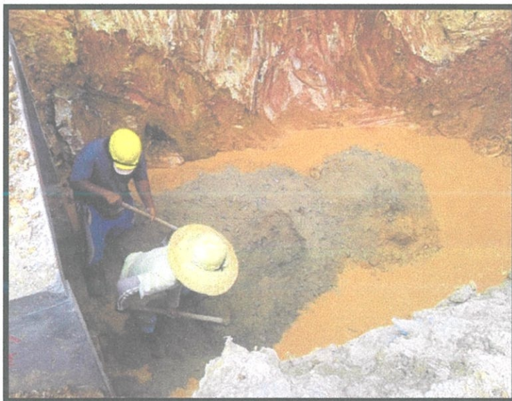
Gambar 3.8: Kerja meratakan crusher run .
