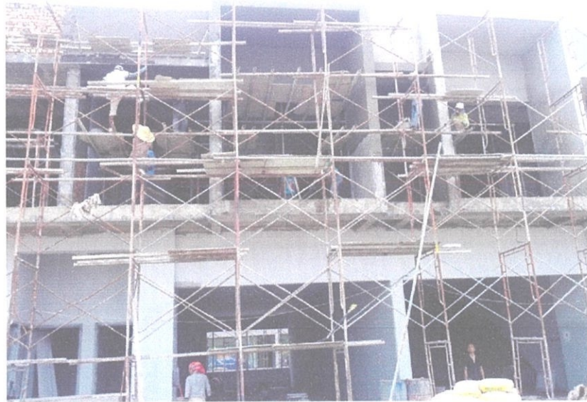
Photo 3.1.3 Worker doing external plastering
