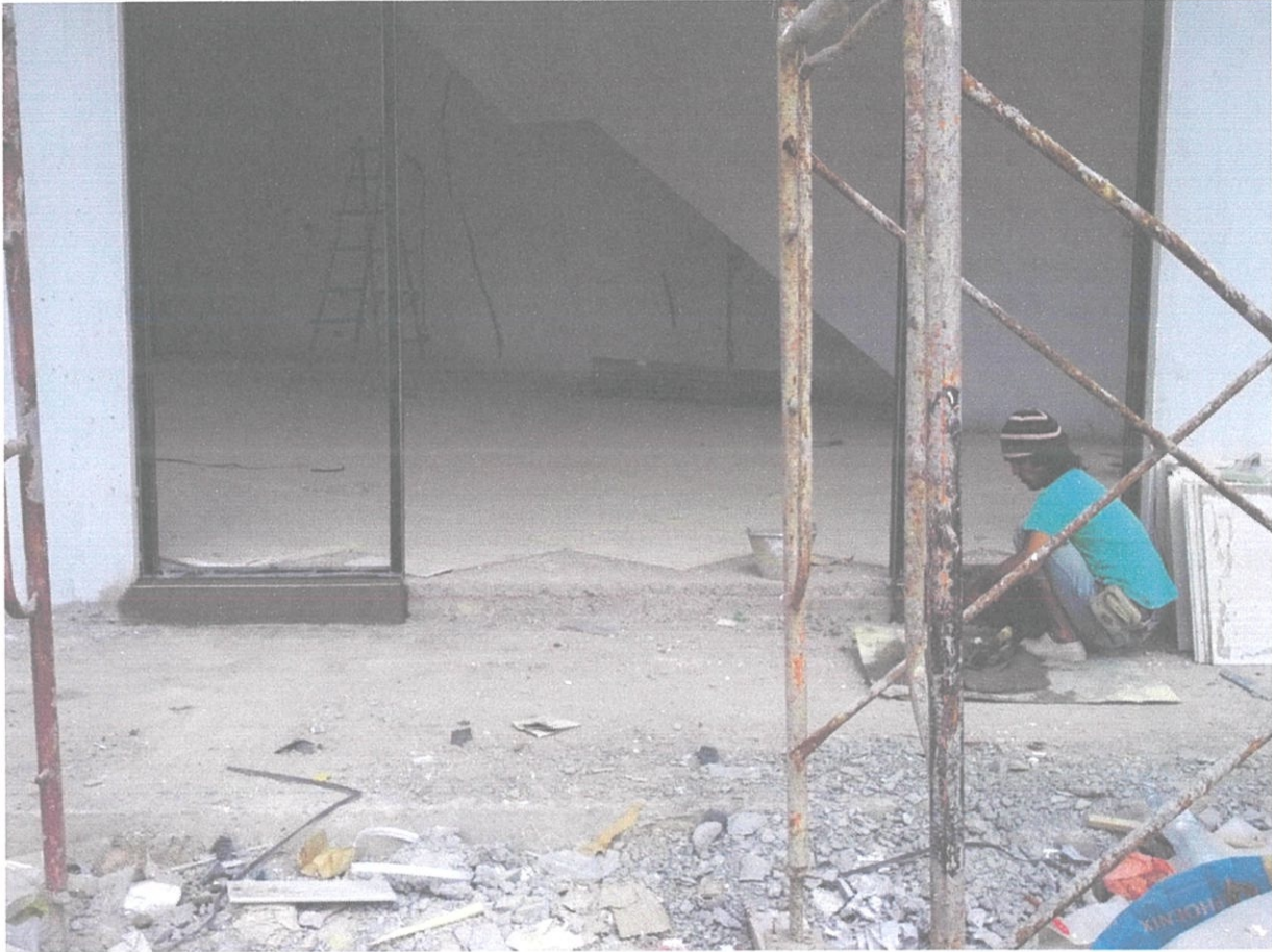
Photo : External plastering in-front main door
