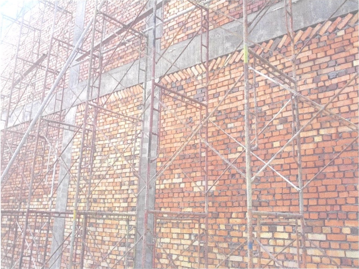
Photo : External wall before plaster
