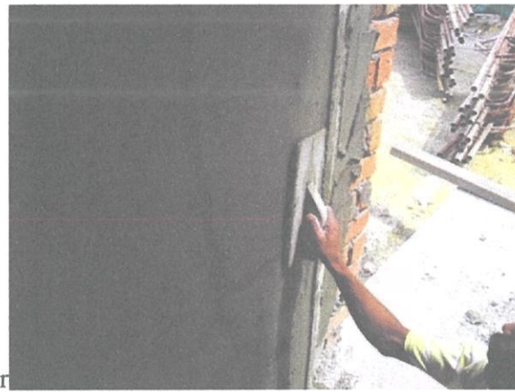
Photo 3.1.1 Plastering work
