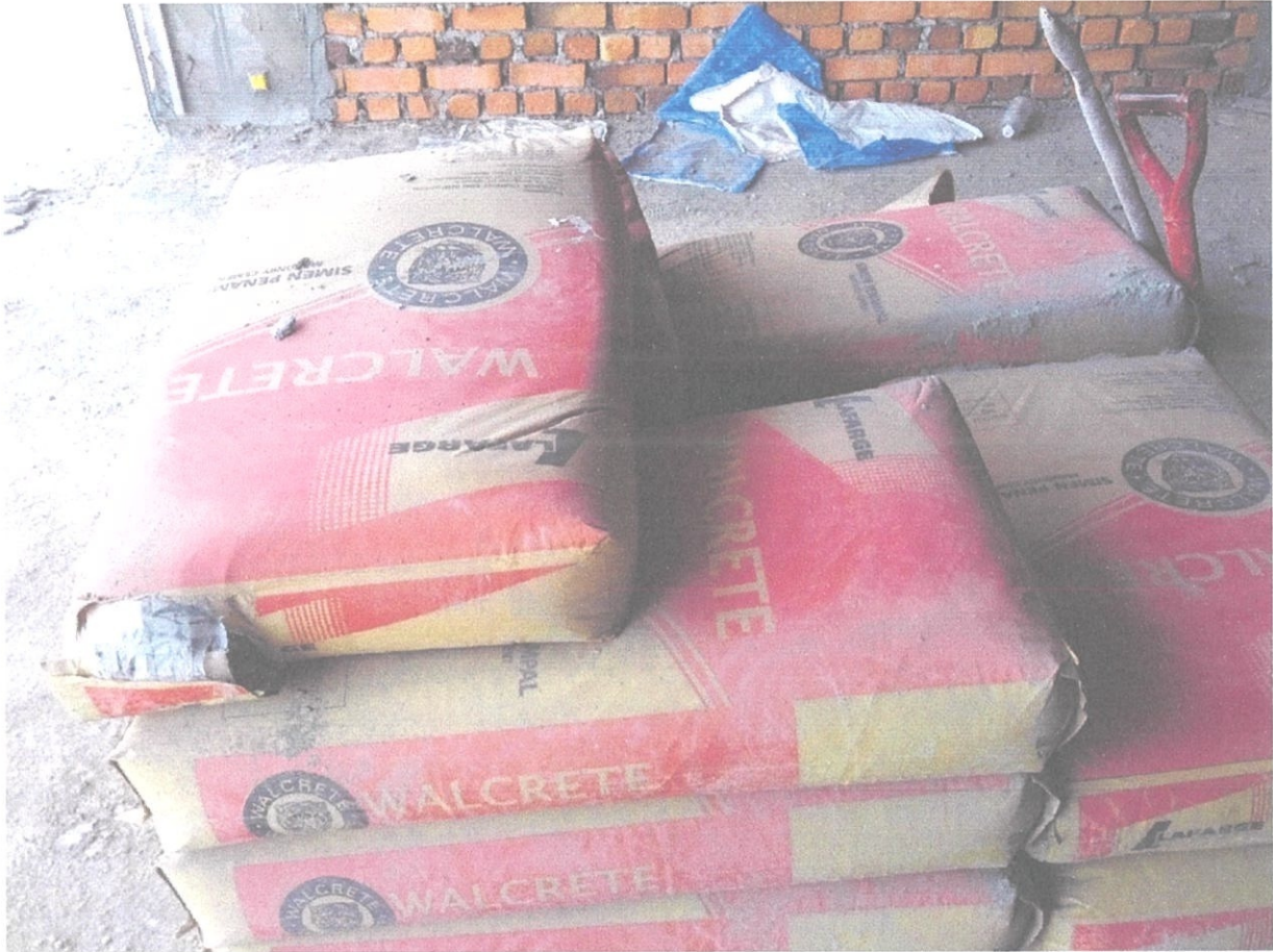
Photo: Walcrete cement is using for the plastering
