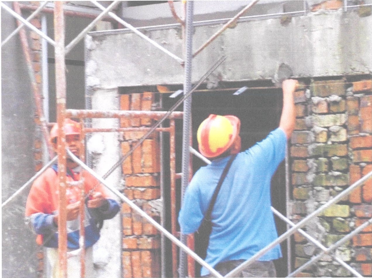
Photo; Marking the thickness of external plastering
