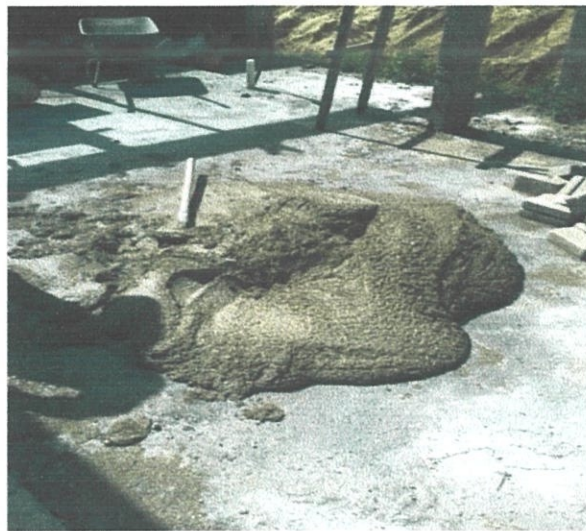
Gambar 3.3 : Bancuhan mortar
