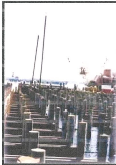
Photo 3.2 The timber piles
