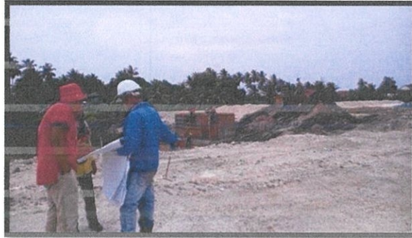
Photo 3.11 Checking the point of piles
