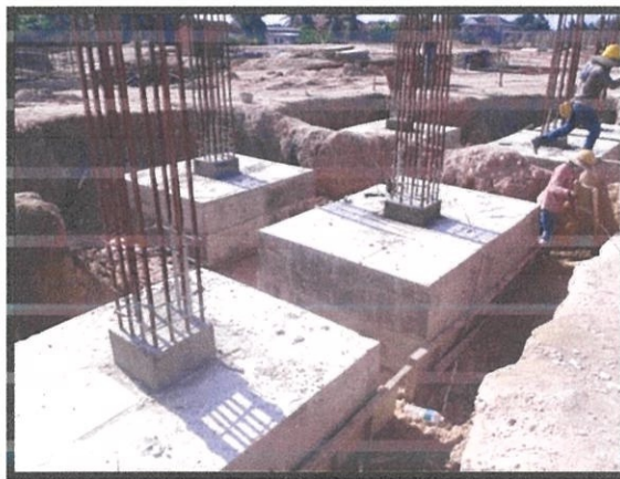
Photo 3.22 The completed pile cap
