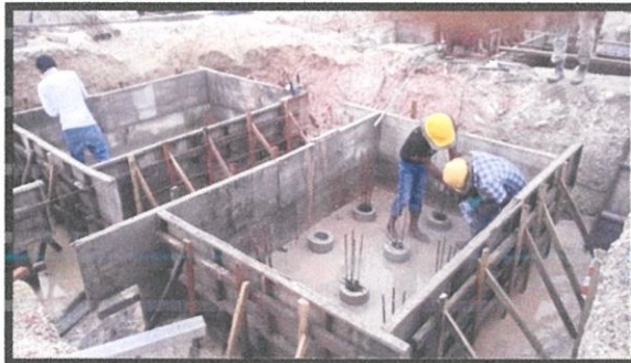
Photo 3.19 Fixing pile cap starter bar
