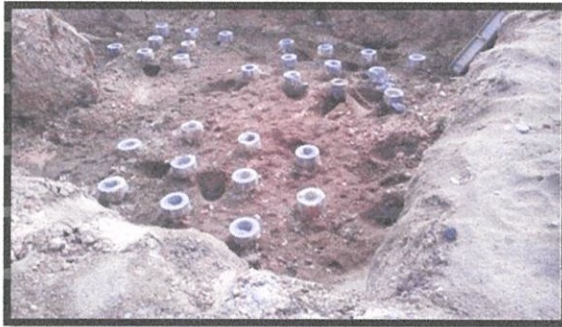
Photo 3.16 Completed cutting off piles
