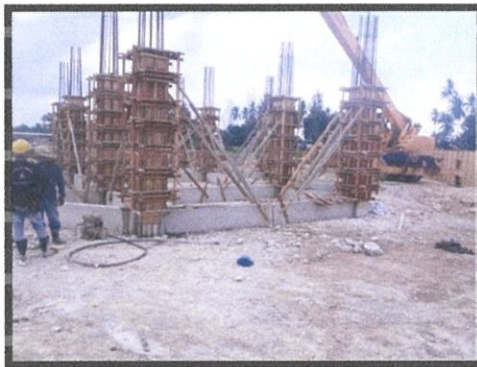
Photo 3.29 Erecting the formwork of column stump
