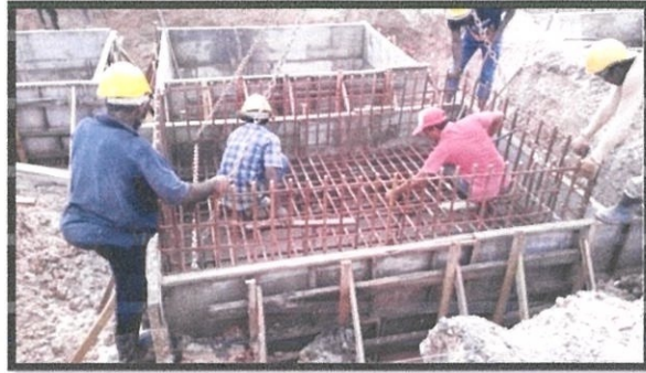
Photo 3.20 Placing the reinforced concrete pile cap into the formwork
