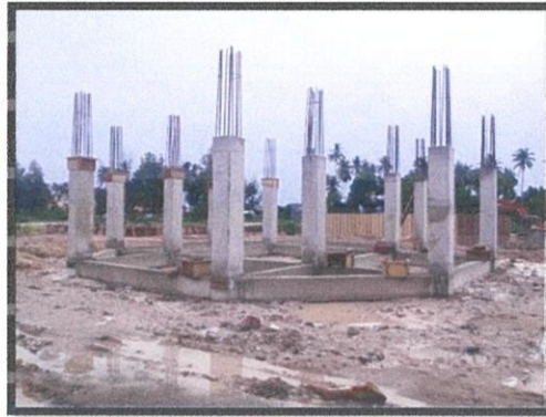
Photo 3.31 The completed column stump
