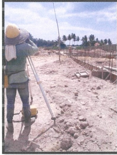
Photo 3.10 Surveying for setting out
