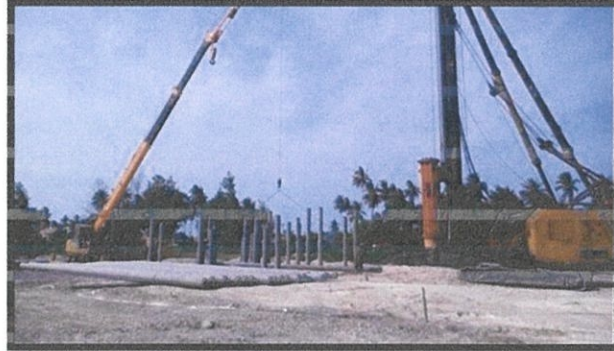
Photo 3.13 Hydraulic hammer used for driven piles into ground
