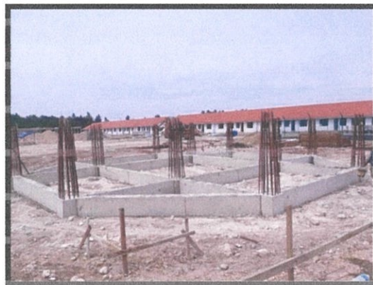
Photo 3.27 The completed ground beam
