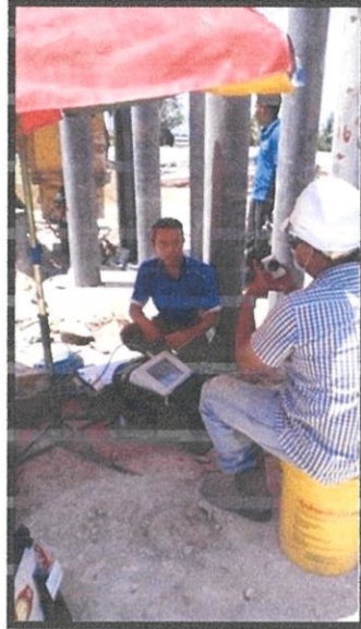
Photo 3.14 PDA test by Geotech Pile (M) Sdn Bhd using CAPWAP software
