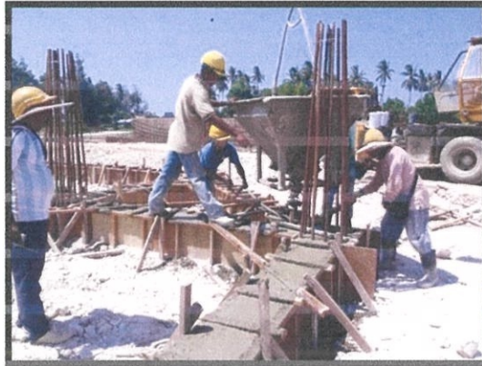
Photo 3.26 Concreting the ground beam
