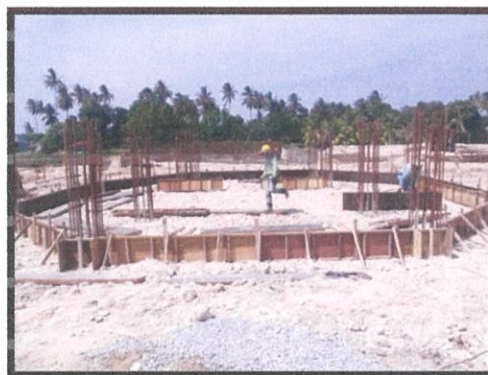
Photo 3.24 The formwork for ground beam being erected
