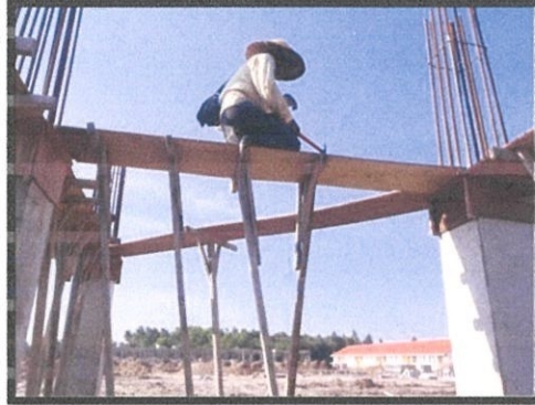
Photo 3.32 The formwork of first floor beam being installed on the columns
