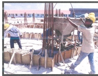
Photo 3.7 Concrete bucket
