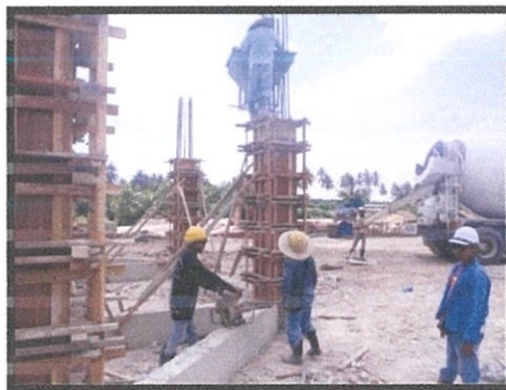
Photo 3.30 The column stump poured with concrete
