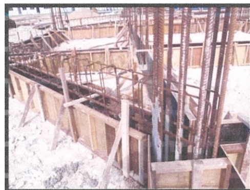
Photo 3.25 Fixing the RC beam into the formwork
