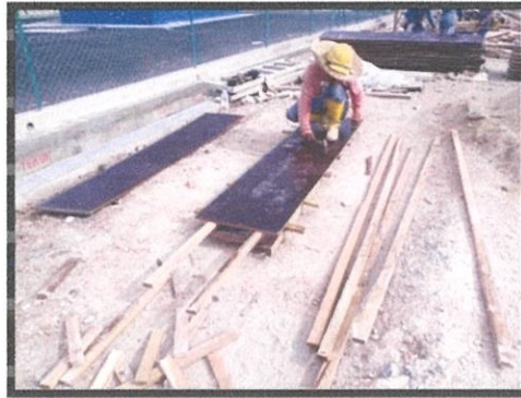
Photo 3.23 Setting up the formwork for ground beam
