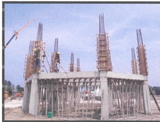
Photo 3.37 The formwork being erected
