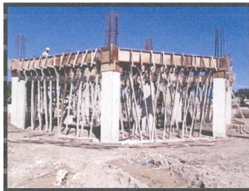
Photo 3.33 The completed formwork for first floor beam
