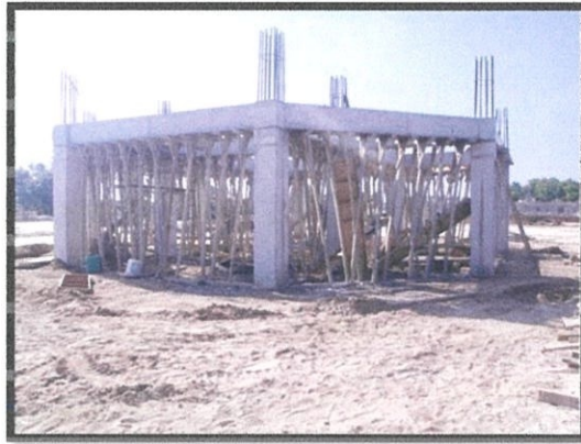
Photo 3.35 The completed of first floor beam
