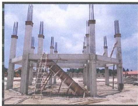
Photo 3.41 RC staircases ready for concrete
