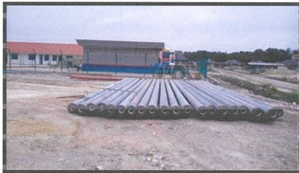
Photo 3.12 Spun piles marked for every feet
