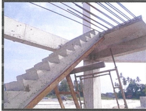
Photo 3.42 The completed RC staircases
