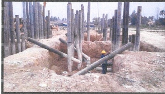
Photo 3.15 Cutting the piles using oxy cutter
