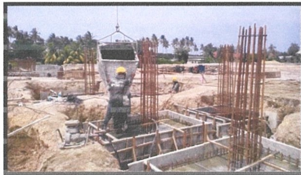
Photo 3.21 Concreting of pile cap
