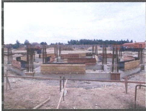
Photo 3.28 Setting up the formwork for column stump
