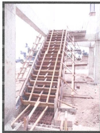
Photo 3.40 Formwork for staircases being erected
