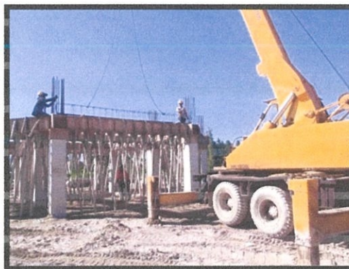
Photo 3.34 Placing the reinforced concrete beam (RC beam)
