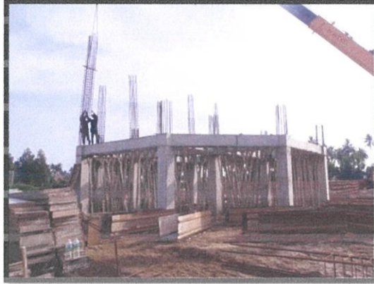
Photo 3.36 Fixing the RC columns
