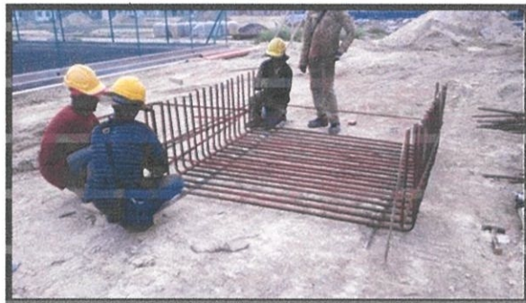
Photo 3.18 Installing the reinforced concrete pile cap
