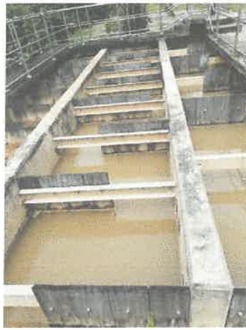
Fig. 55 Flocculation tank
