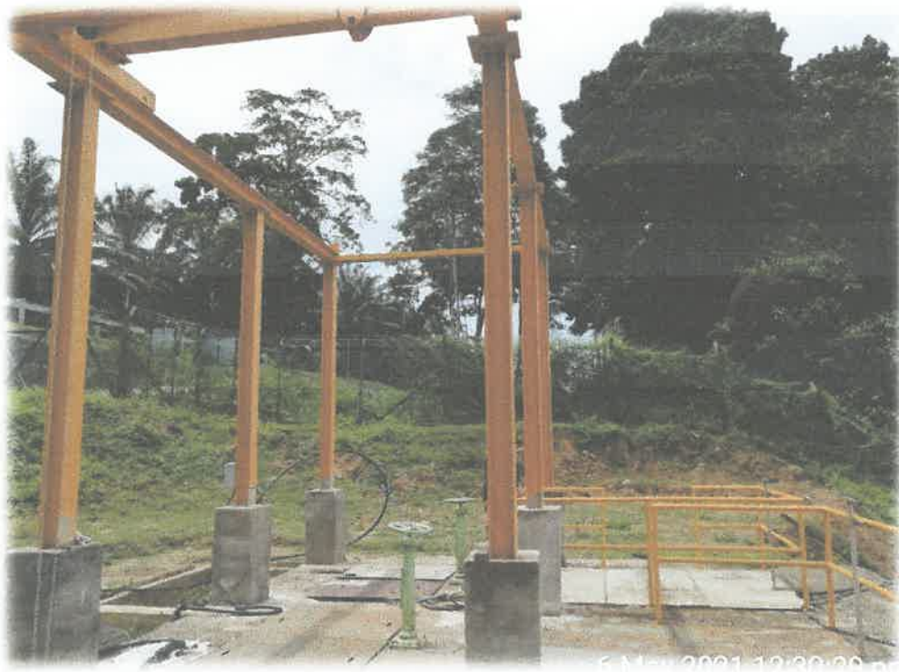
Fig. 49 Activities at May 6, 2021
