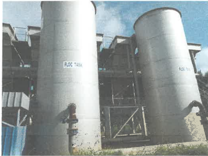
Fig. 58 Flocculation tank
