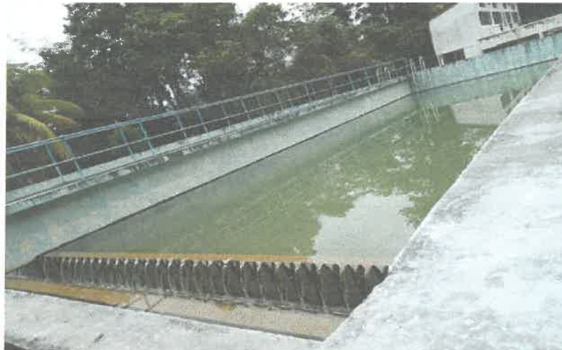
Fig. 56 Sedimentation tank
