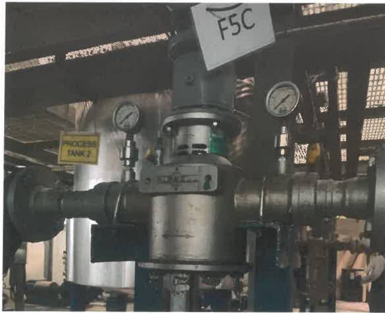
Figure 14 Cleaning the strainer
