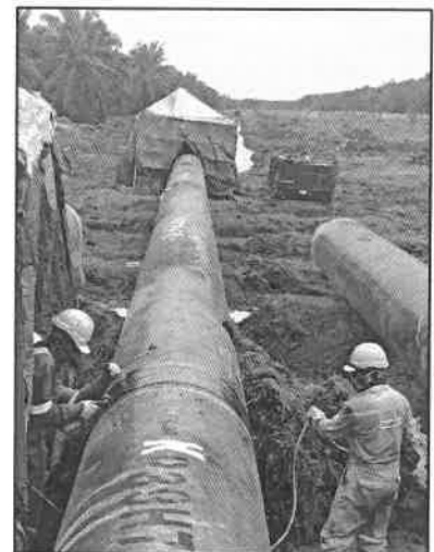
Field Joint Coating (FJC)
