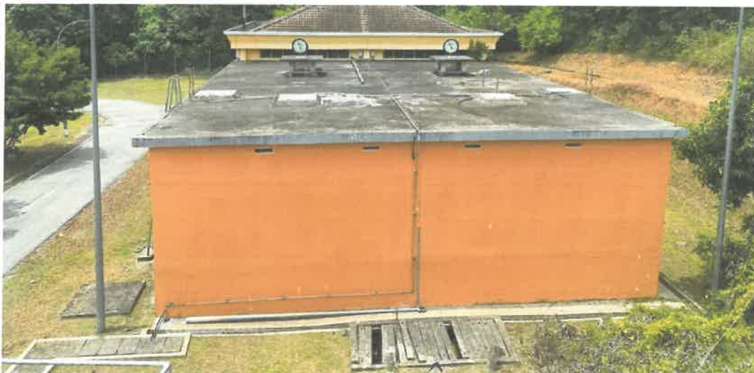
Figure 3.9.1 Clear Water Tank in Titi Water Treatment Plant
