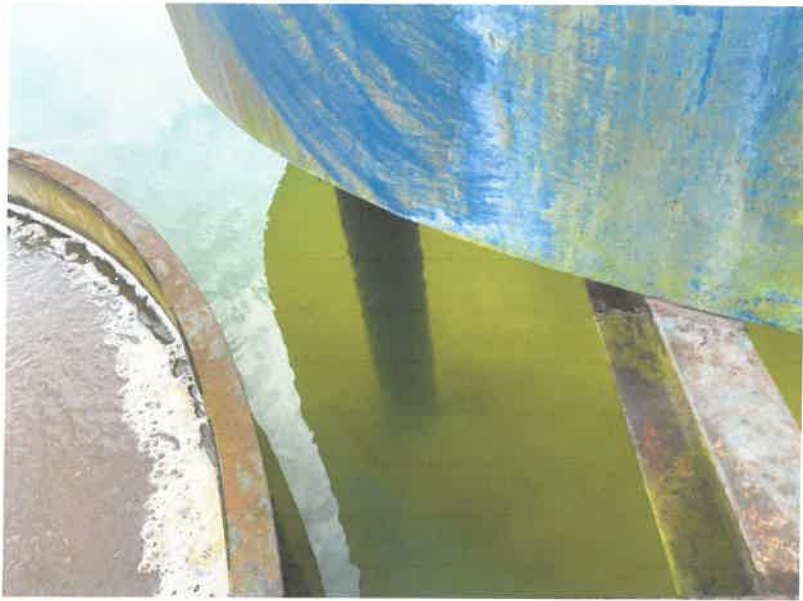
Figure 4.5.8 Formation of sludge blanket
