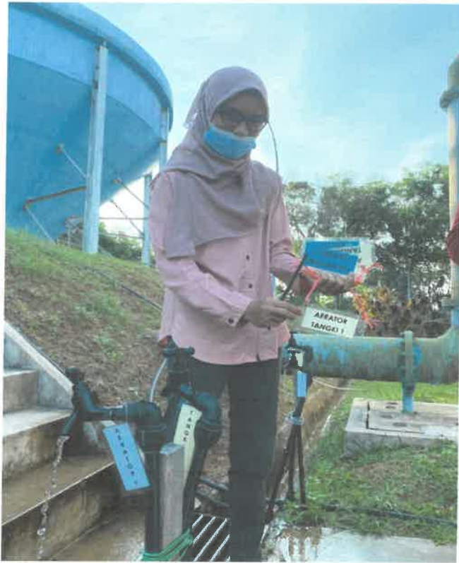
Figure 4.5.63 Tagging water sample pipe
