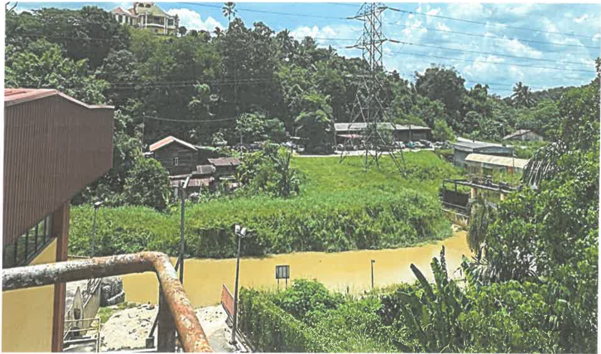
Figure 3.1.1 Intake of Kuala Pilah Water Treatment Plant
