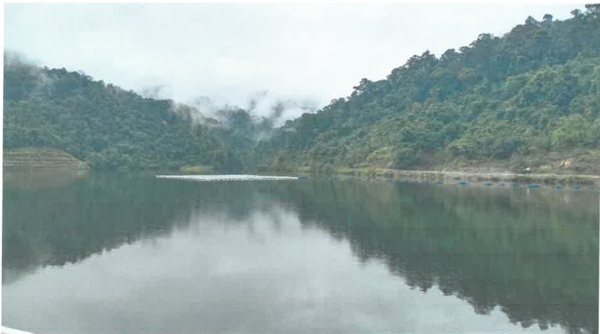
Figure 3.1.2 Intake of Pedas Baru Water Treatment Plant
