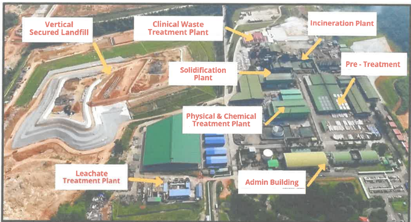
Figure 1.1: Overview of Waste Management Centre (WMC)
