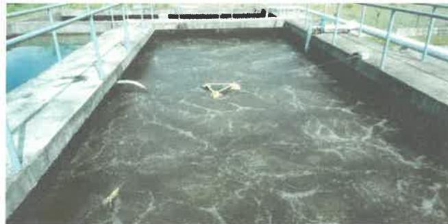
*Figure 2.5 Aeration Tank of the Wastewater Treatment System at Halal Abattoir Complex*
