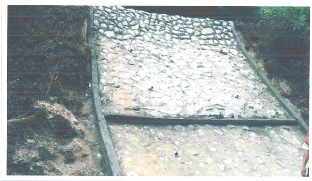
Figure 3.3.3.1: Rubble pitching that has been done at slope area.
