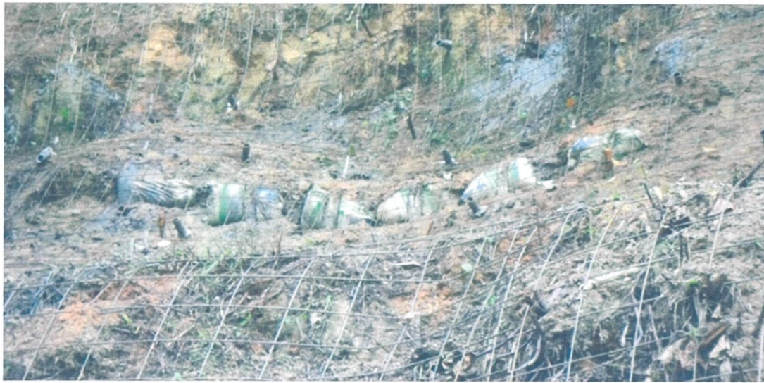
Figure 3.3.5.1: Reinforcement bar on the slope surface
