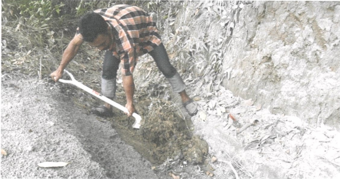
Figure 3.3.2.1: Removal of loose materials from slope
