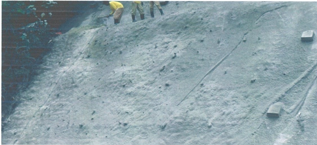
Figure 3.3.6.1: Slope has been sprayed by gunite machine Photo credit: Redza Zamani (2011)
