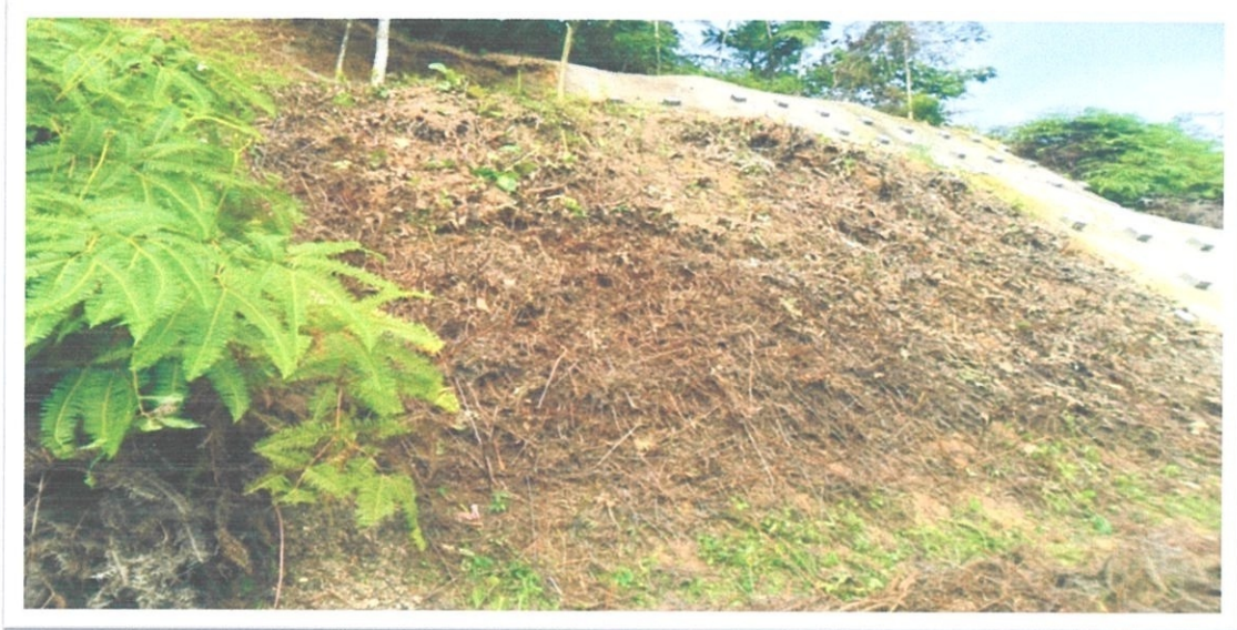
Figure 3.3.1.1: Slope area has been cleared.
