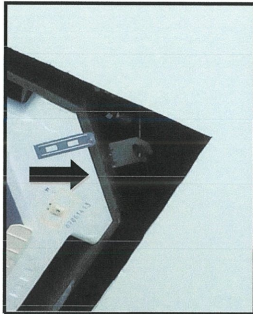
Photo 3.24 screw the cassette unit
