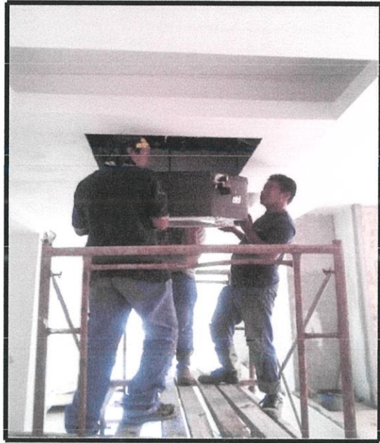
Photo 3.23 lifting cassette unit
