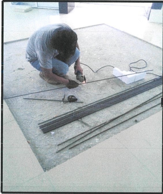
Photo 3.21 cutting steel rod
