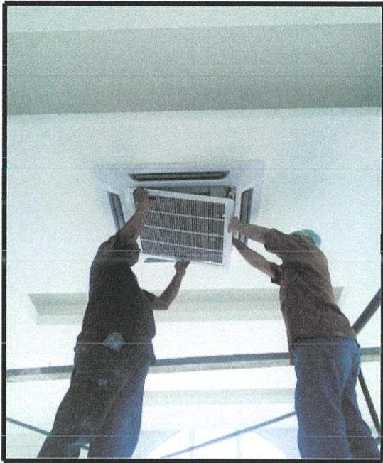
Photo 3.27 install filter
