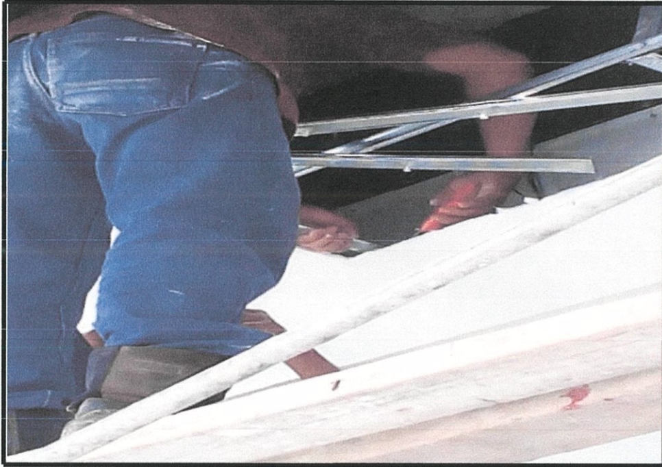
Photo 3.20 removed frame ceiling
