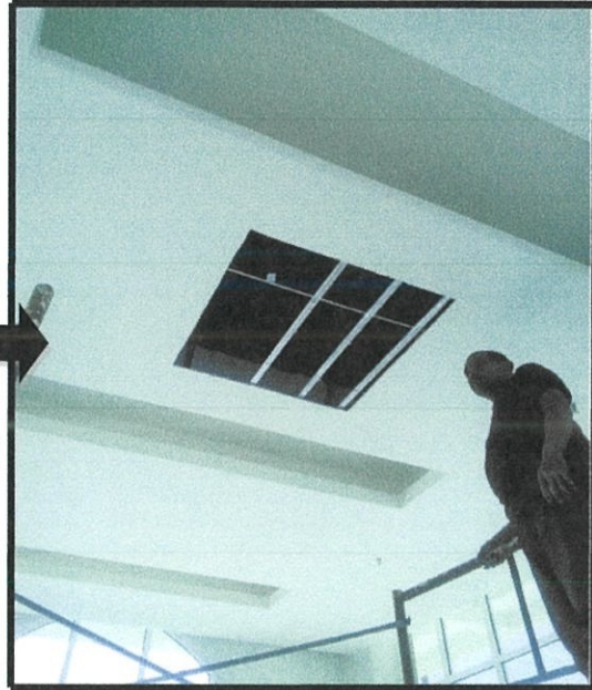
Photo 3.19 removed frame ceiling
