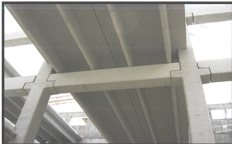
Gambarfoto 3.11: 'Double-Tee Slab'
