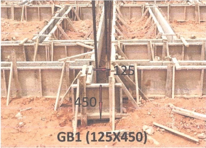
Figure 3.14 Measurements of Formwork
