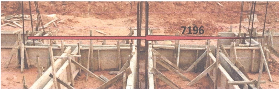
Figure 3.15 Shows the length of GB1 for concreting
