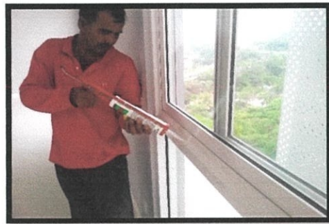
Photo 3.5 The worker replaces a new silicone at living area
