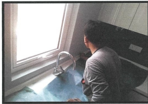
Photo 3.8 Worker replace the silicone sealant
