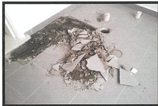
Photo 3.12 Ceramic tiles damages
