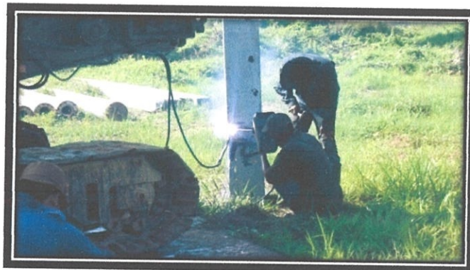
Photo 3.9: Welding the pile for the connect
