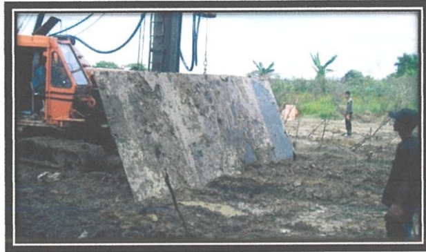
Photo 3.16: Plate was use to easy move on
