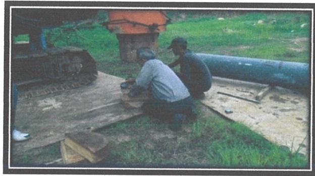
Photo 3.5: Lining the wood at the piling machine
