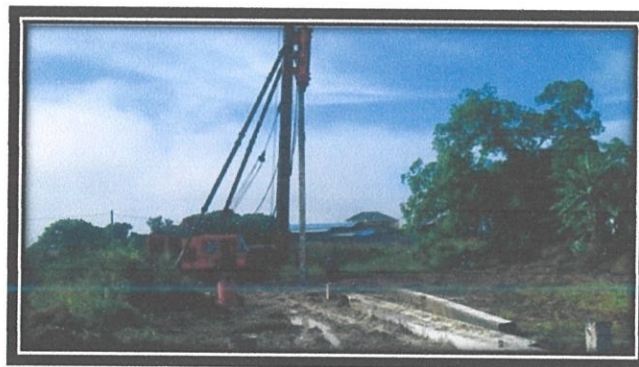
Photo 3.6: Piling machine drop the pile
