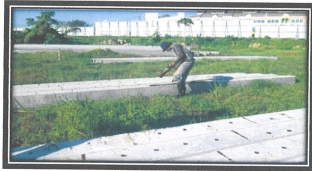
Photo 3.4: Marking the pile by using paint
