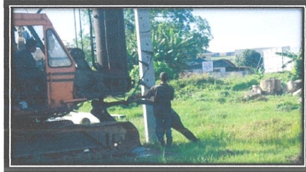
Photo 3.7: Adjust the pile for to straight
