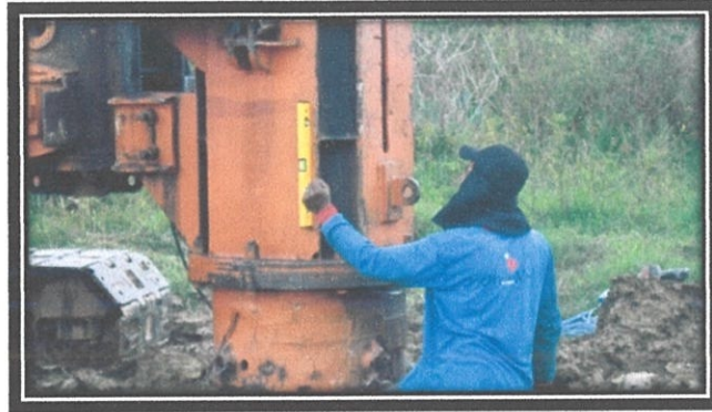
Photo 3.22: Measure the pile
