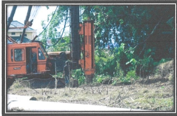
Photo 3.18: Piling machine show drop of pile
