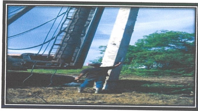
Photo 3.8: Measure the pile use sprit level
