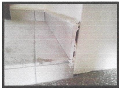
Photo 2.4: Hollowness at the tiles joint.
