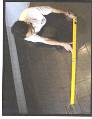
Figure 3.5: Inspecting falls in wet areas.
