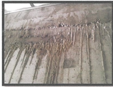
Photo 2.5: Dirtied wall surface with the excessive concrete.
