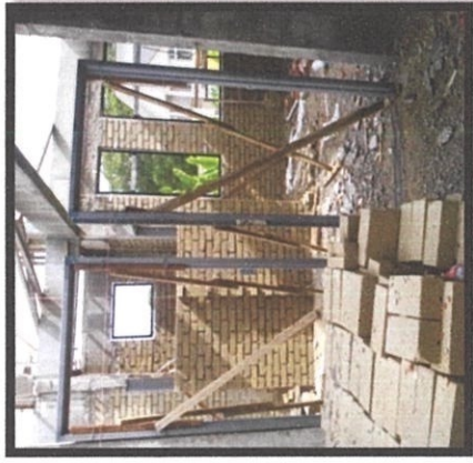
Photo 4.2: Timber as the temporary supporter of frame.
