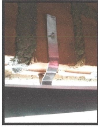
Photo 4.2: Timber as the temporary supporter of frame.
