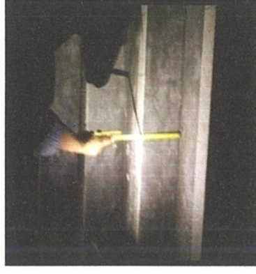
Photo 3.1: Checking the angle between a column and wall.
