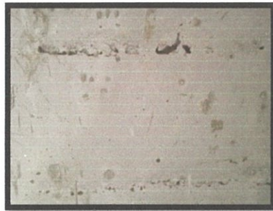
Photo 2.3: Honey comb on the concrete.
