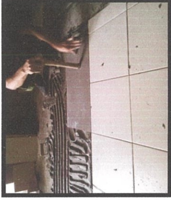
Photo 3.7: Tap the tile by using a rubber mallet.
