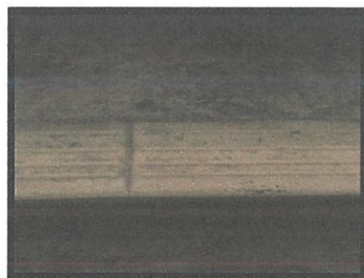
Photo 2.7: The suitable material of nosing (non-slip tile).
