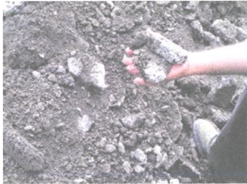
Photo 3.3 Concrete have to be broken up.
