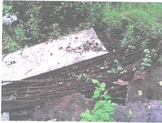
Photo3.11 Reinforcement bar on open area.
