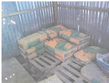
Photo 3.22 Cement lined to avoid contact with water.
