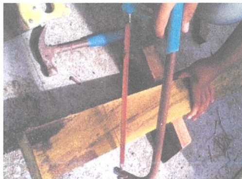
Photo3.17 Wrong equipment used.
