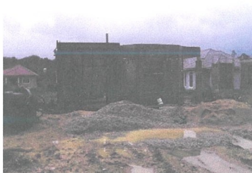
Photo 3.6 Aggregate mixed with mud.
