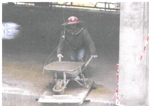
Photo3.2 Concrete transport by wheelbarrow.
