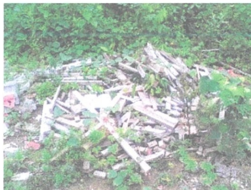
Photo3.20 Wood cannot be used because wrong when cutting work.
