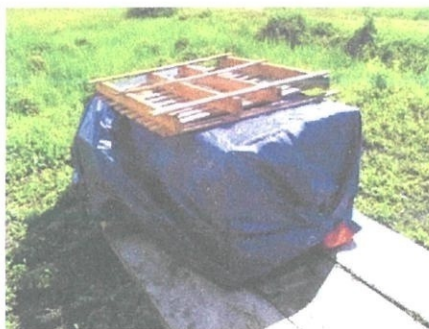
Photo 3.23 Tiles fully cover.
