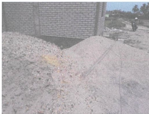
Photo 3.8 Sand placed near with work area.
