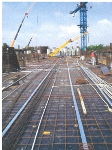
Photo 3.14: Installing of Stressing Anchirages to Formwork
