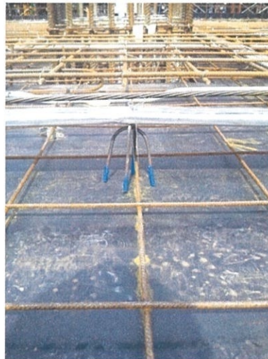
Photo 3.17: Installation of Beams and Slab Tendon.
