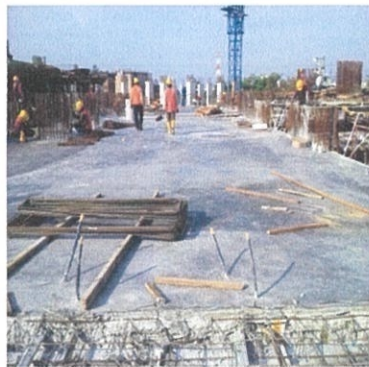
Photo 3.24: Patching of Ftressing Recess.
