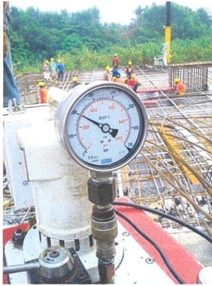
Photo 3.22: Control of Stressing Operations.
