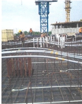
Photo 3.16: Installation of Beams and Slab Tendon.
