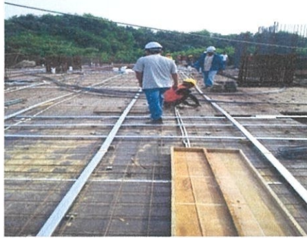
Photo 3.18: Checking of Tendon Profile.
