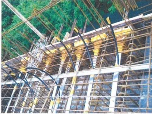
Photo 3.5 : Anchorages Recess.
