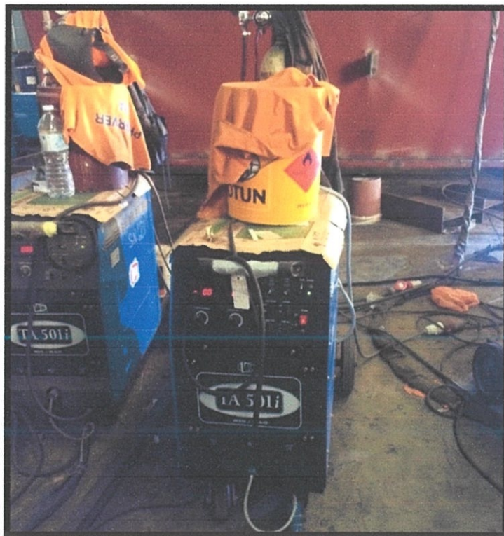
Photo 3.11 Flux Core Machine for welding works.
