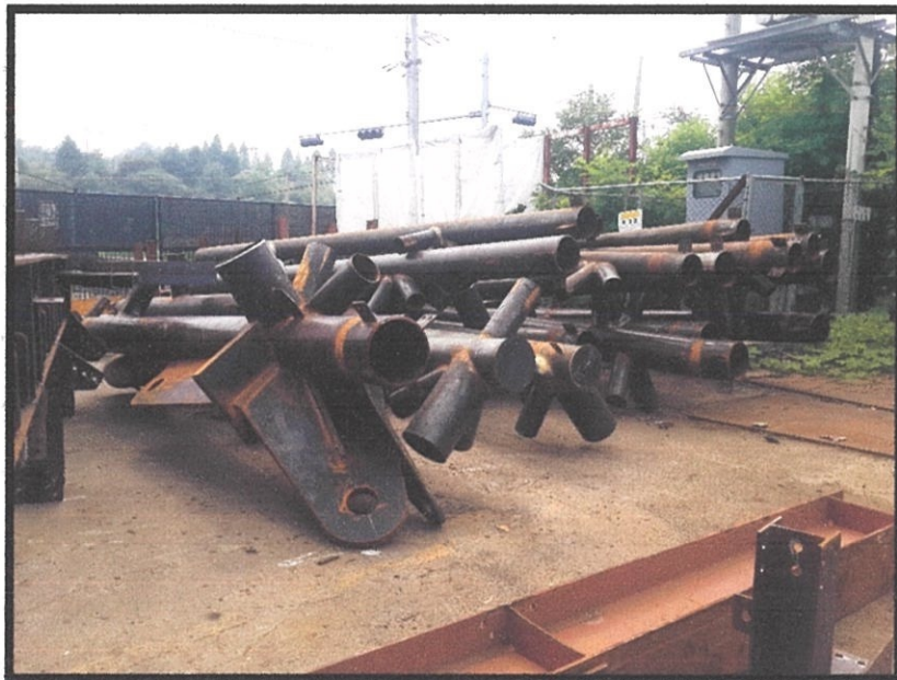
Photo 3.2 Material lay down in the factory.
