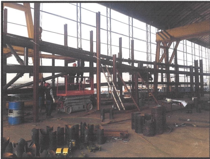
Photo 3.6 A steel free from bending and twist being placed on the jigs.
