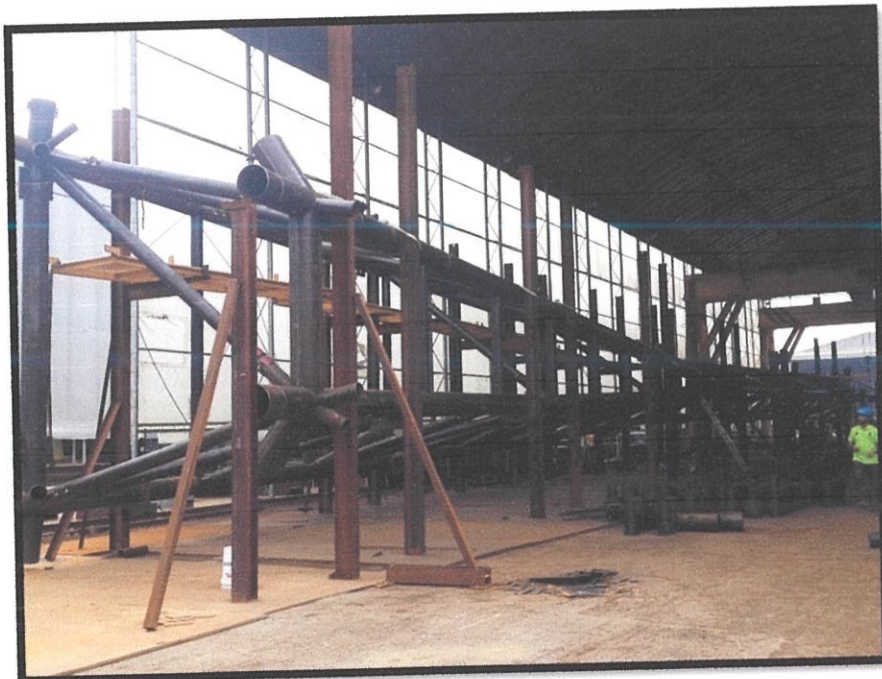
Photo 3.8 Assembly area for the steel trusses.
