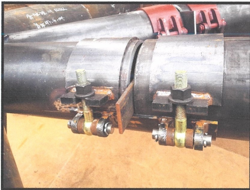
Photo 3.10 A visual of root gap prior to welding process.
