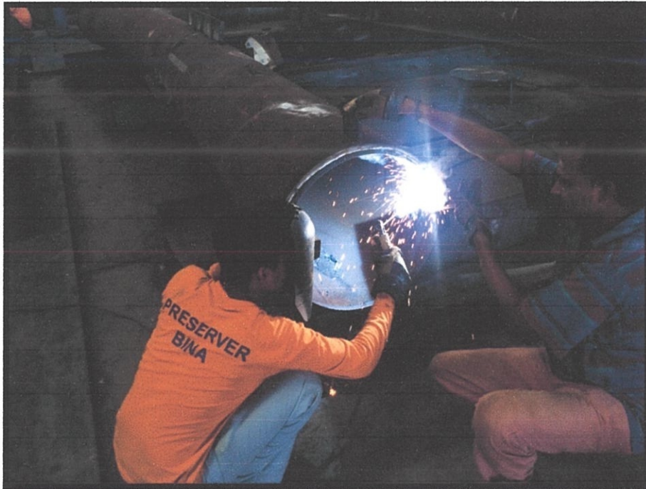
Photo 3.13 Welding process made by the workers.
