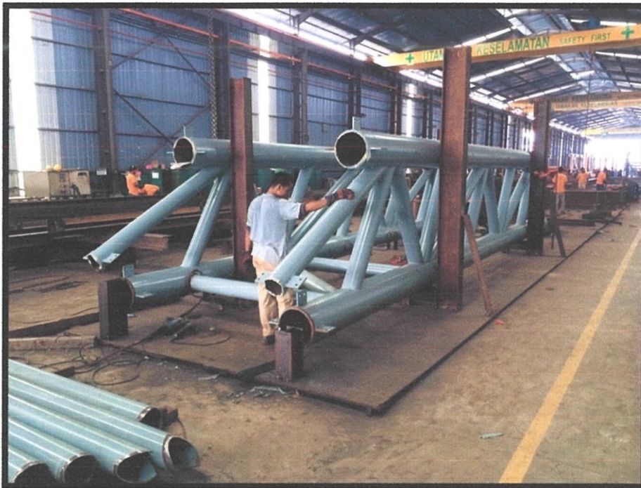
Photo 3.17 Steel trusses after paint.
