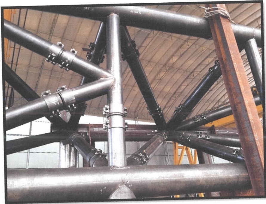
Photo 3.7 Preassembled steel trusses.
