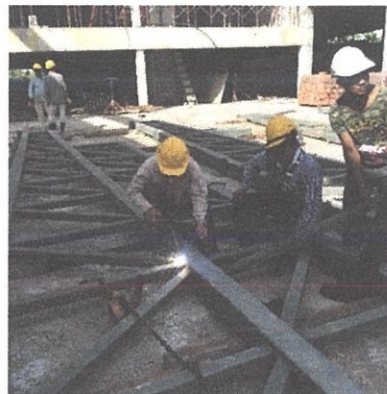
Photo 3.3: Assemble the mild steel truss
