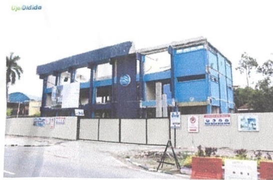
Photo 3.1 Bangunan SADA before renovation
