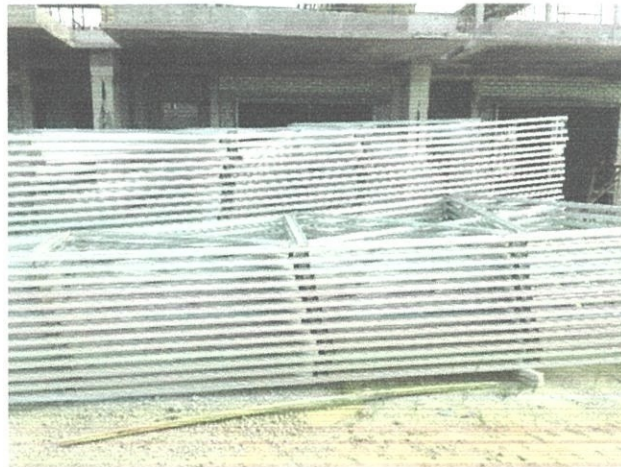
Photo 3.12: Trusses being stack up.
