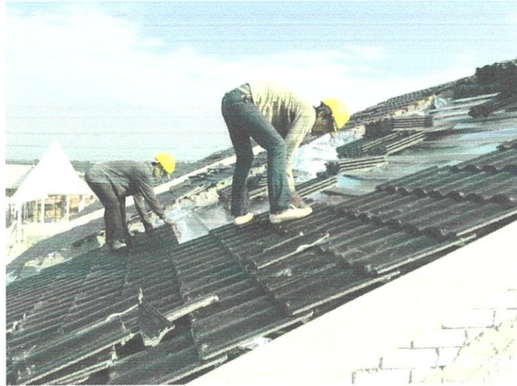
Photo 3.23: Workers install the roof tiles.
