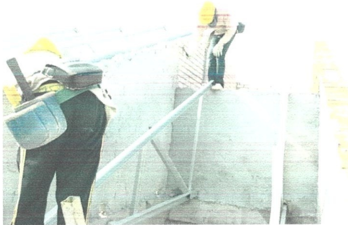
Photo 3.16: Workers align the trusses.
