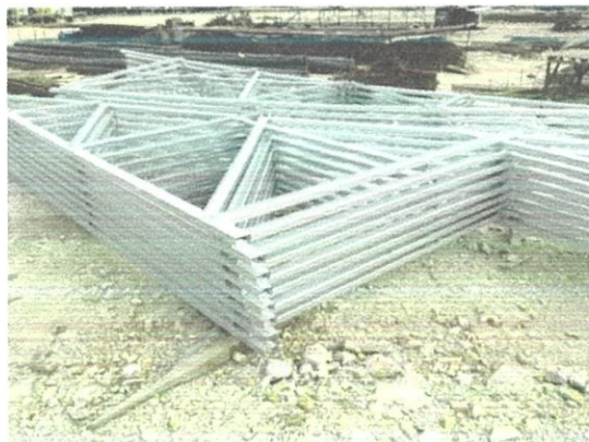
Photo 3.6: Subsequent of trusses.
