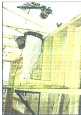
Figure 3.3: A worker installing roof trusses from an interior bracket scaffold.
