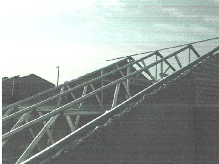
Photo 3.17: Trusses being arranged.
