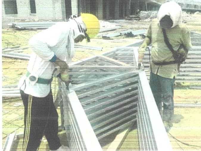
Photo 3.9: Workers fasten the apex joint.
