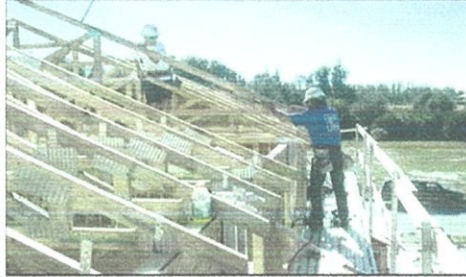
Figure 3.4: Workers using an exterior bracket scaffold to install roof trusses.
