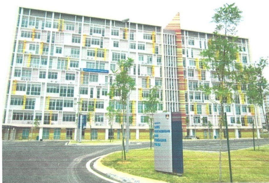
Photo 2.6 : Front elevation of Administration Office, UITM Seremban.
