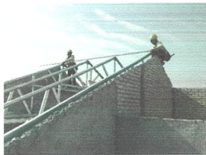
Photo 3.4 : the same 2 workers connect the trusses to the roof beam.
