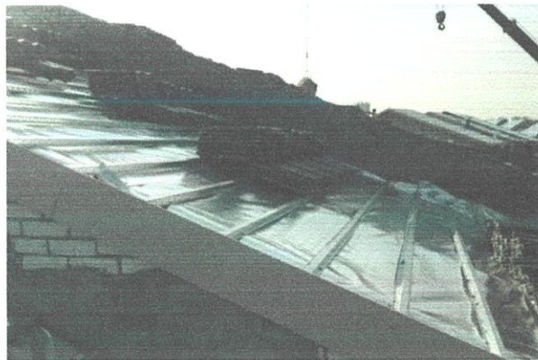
Photo 3.22: Roof tiles before the installation.
