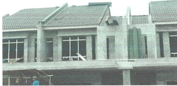
Photo 3.25: Trusses are fully installed.
