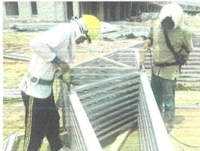
Photo 3.2 : 2 Workers connect the c-channel to become a trusses.
