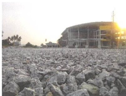
Photo 3.5: crusher run after compacted
