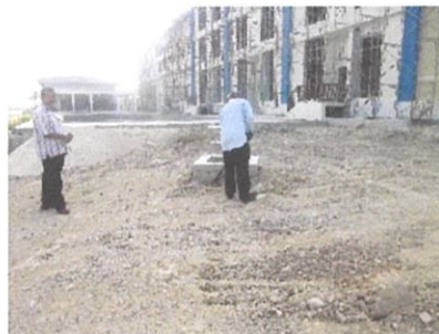
Photo 3.1: A worker doing clearance job
