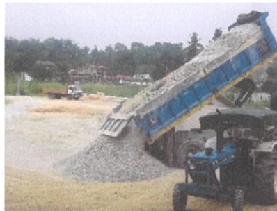
Photo 3.2: crusher run is delivered by a huge amount
