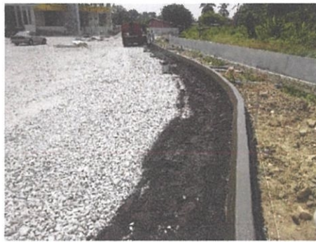
Photo 3.12: Pipe is directly installed after kerb had laid
