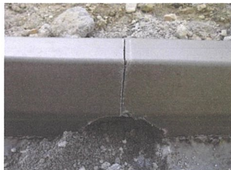
Photo 3.9: Hole and line made at every 5 metre kerbs
