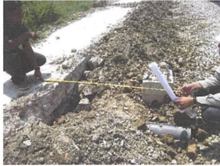
Photo 3.11: Measure the length to install the pipe between kerb and drain
