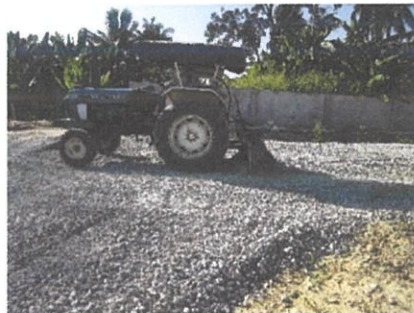
Photo 3.4: back pusher is laying the crusher run
