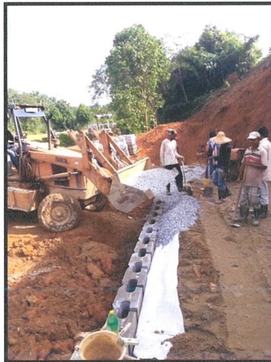
Photo 3.19 Insert aggregate 20mm
