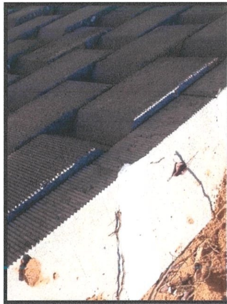
Photo 3.20 Capping top wall
