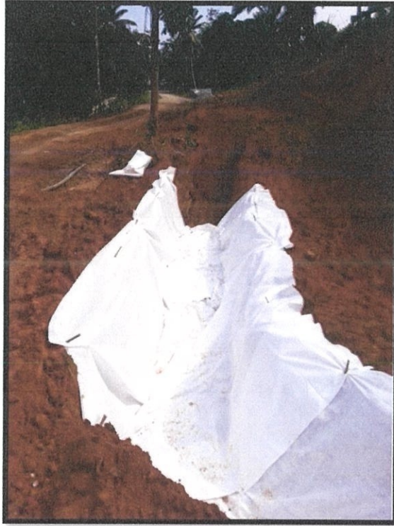
Photo 3.10 Insertion of Geotextile into the base
