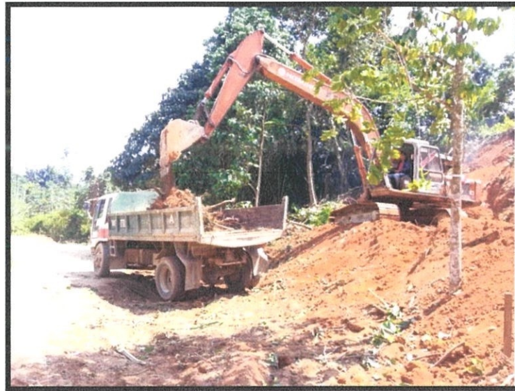
Photo 3.6 Loading of waste on truck
