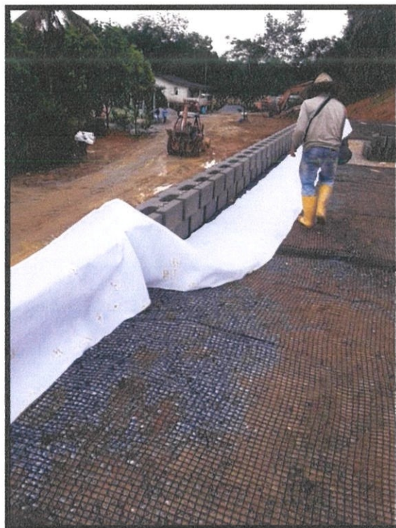
Photo 3.17 Insert geotextile
