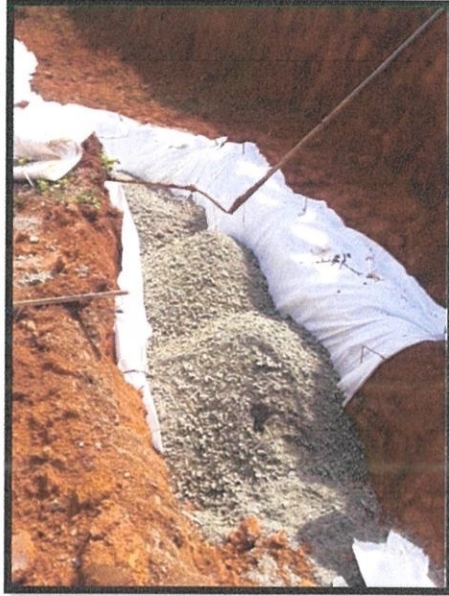
Photo 3.11 Insert crusher run
