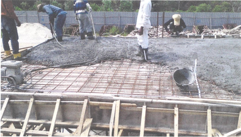
Photo 3.8 : The concreting process of first floor slab and first floor beam
