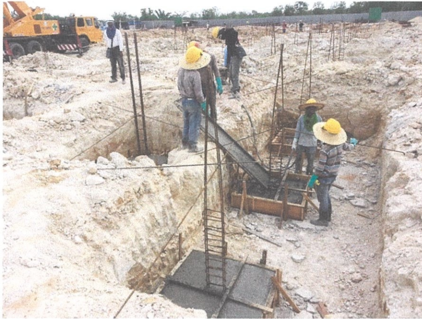
Photo 3.2 : The concreting process of pad footing
