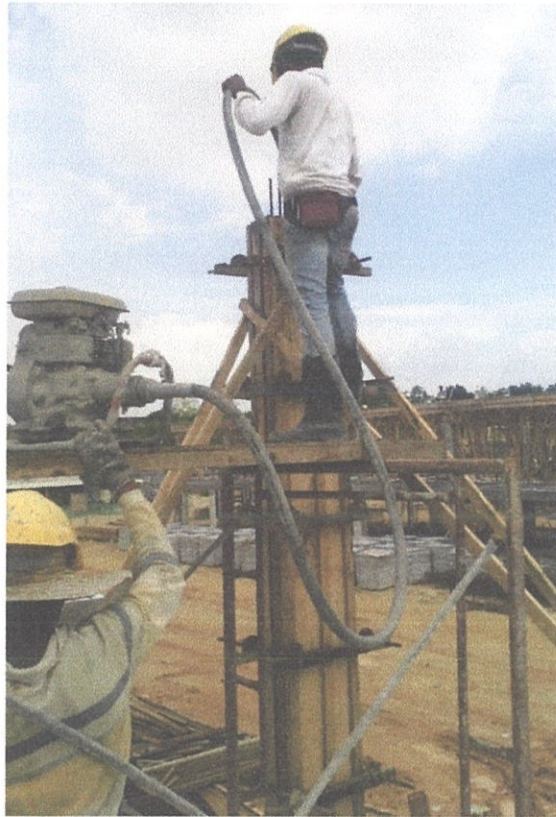
Photo 3.9 : The vibration work while concreting the column
