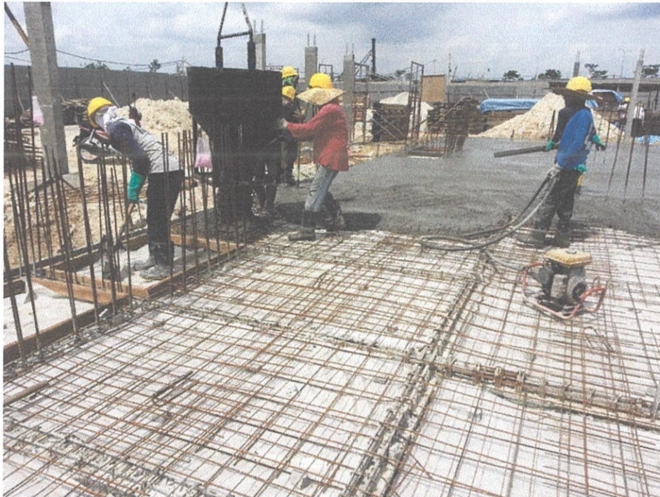
Photo 3.7 : The concreting process of ground floor slab
