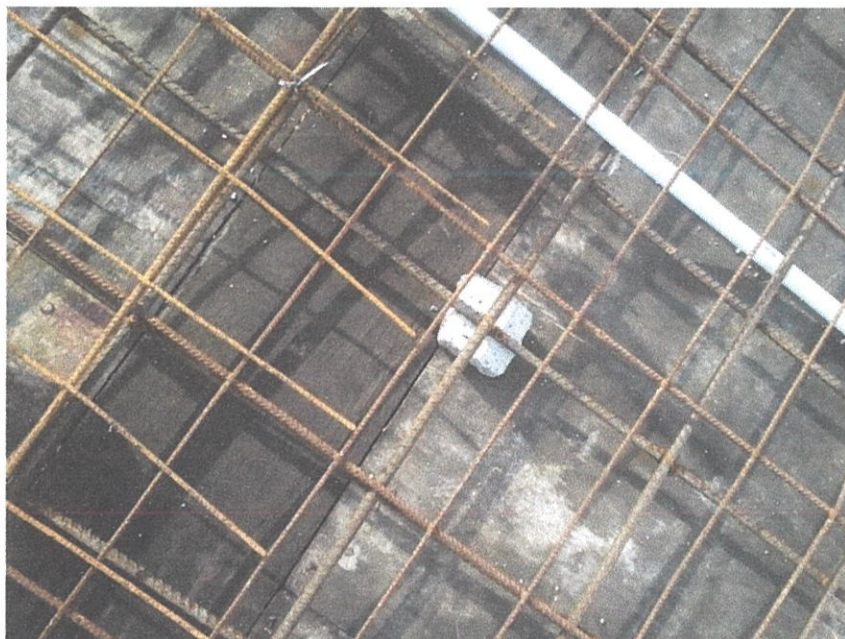
Photo 3.6 : The example of spacer that placed at the bottom of BRC
