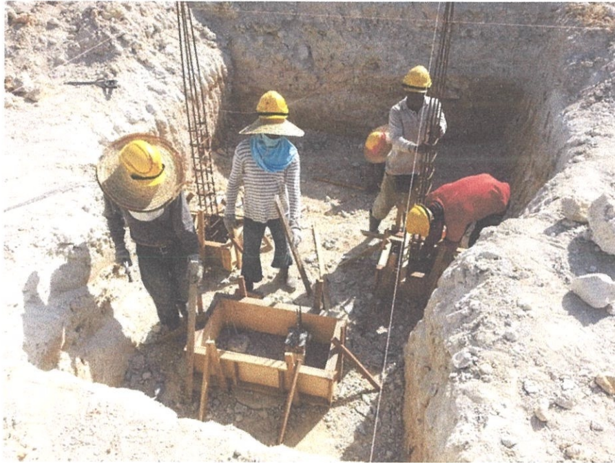
Photo 3.1 : The installation of pad footing formwork
