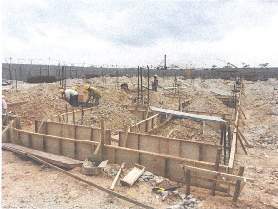
Photo 3.3 : The installation of ground beam formwork
