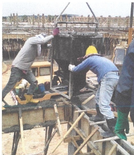
Photo 3.10 : Concreting of roof beam
