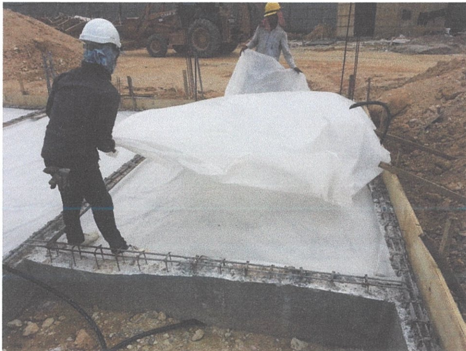
Photo 3.5 : Process of laying a Damp Proof Membrane (DPM)
