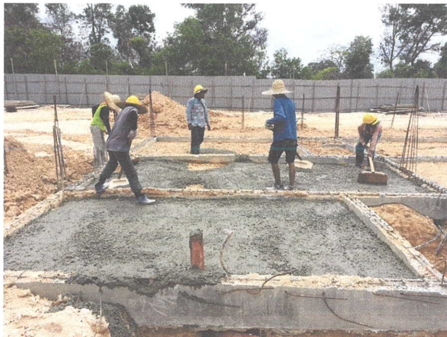
Photo 3.4 : The concreting of lean concrete in the slab
