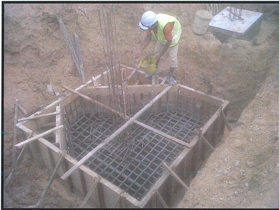
**Picture 3.10** Pile cap timber formwork
