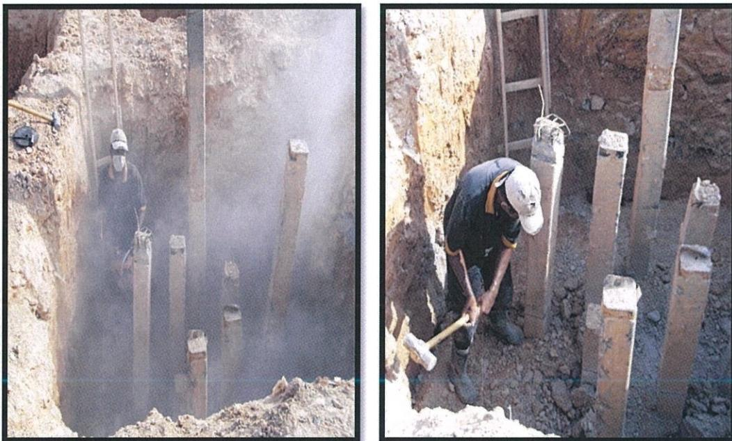
**Picture 3.9** Pile cutting work
