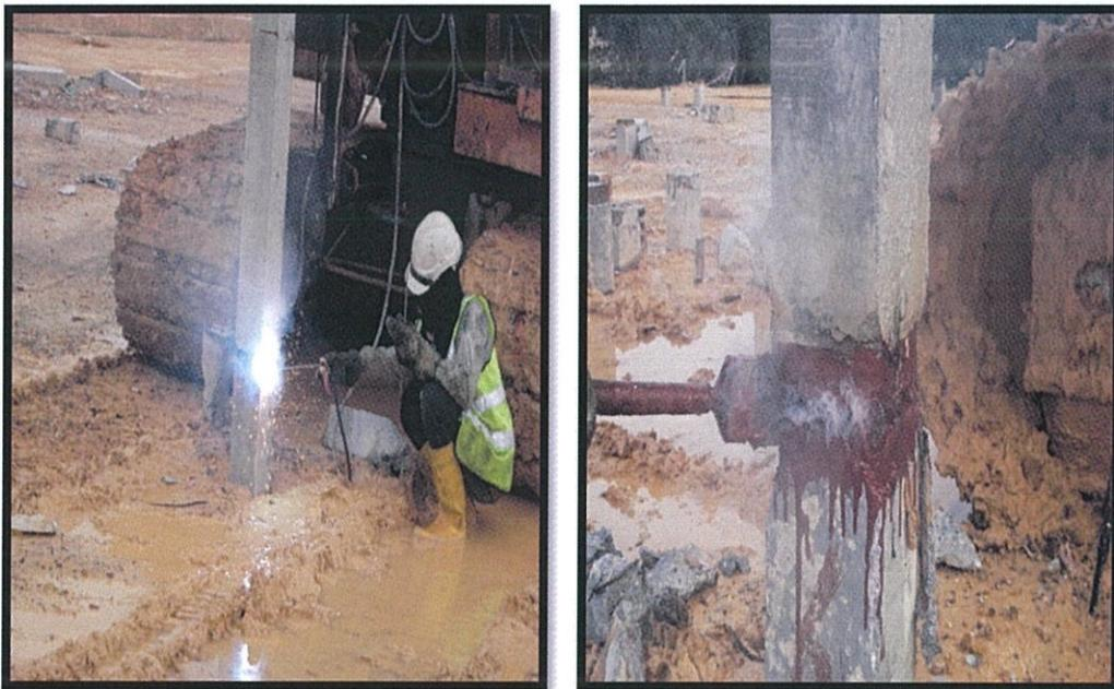
**Picture 3.6** Pile welding and coating
