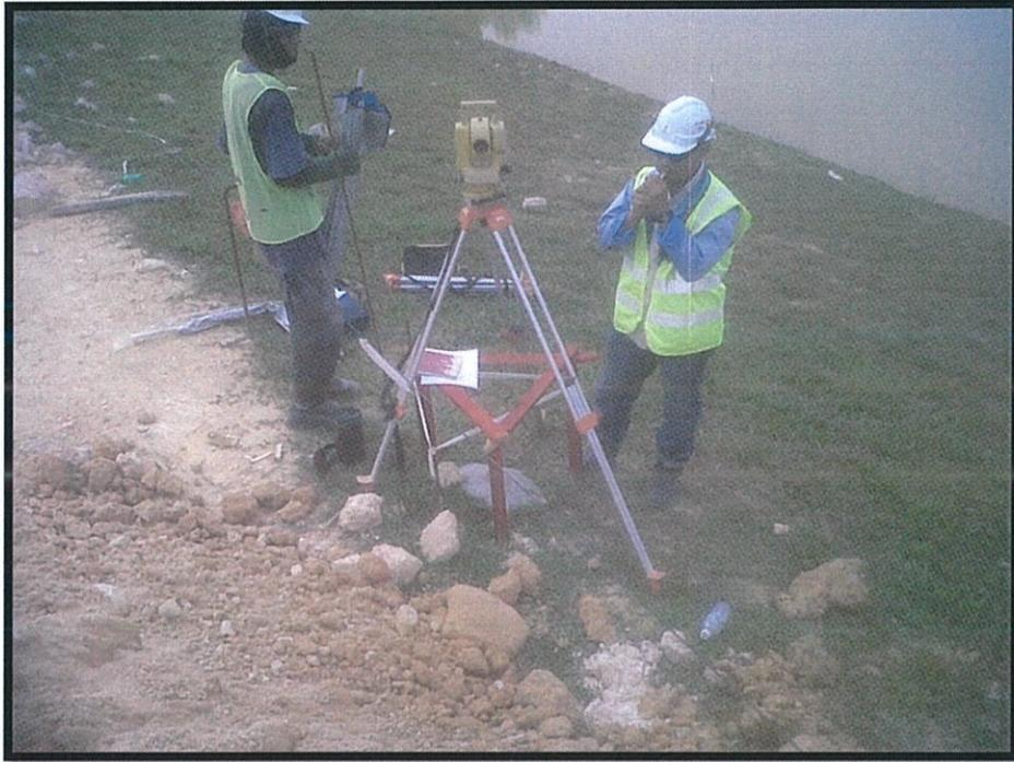
**Picture 3.3** Setting out the pile position
