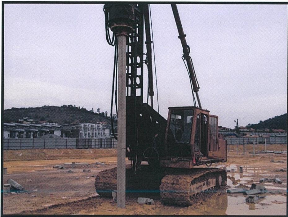
**Picture 3.5** Drive pile into the ground
