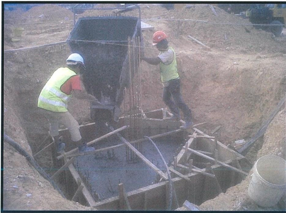
**Picture 3.12** Pile cap concreting work
