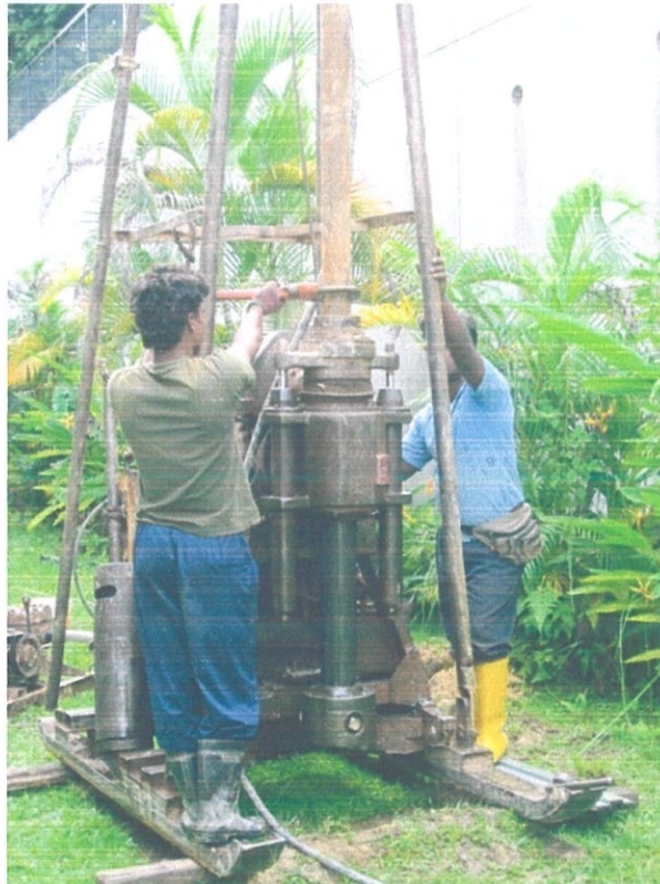
Figure 4.6: Installation of the machine.
