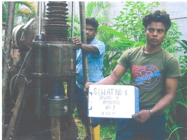
Figure 4.7: Work can start if all the preparation is complete.
