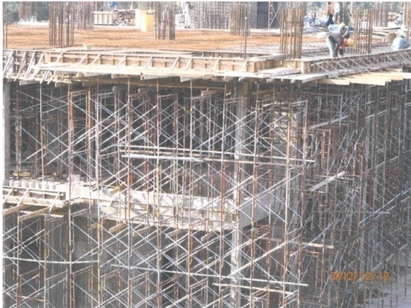
Picture 3 : Frame scaffolding
