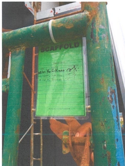
Picture 7 : Safety Tagging of Scaffolding
