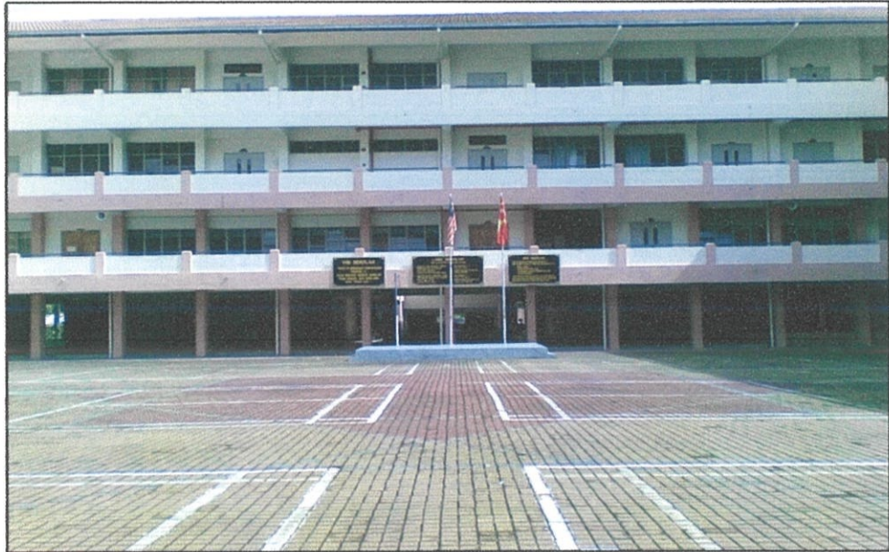
Figure 2.4: Secondary school at section 27.
