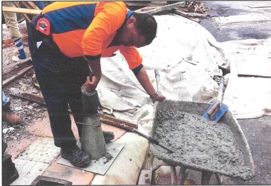
Photo 3.4: The frustum is fill with concrete.
