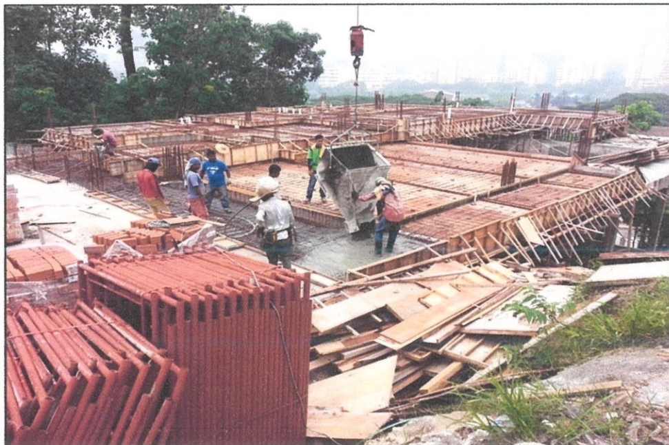
Photo 2.1: The concreting is in progress on ground floor level.
