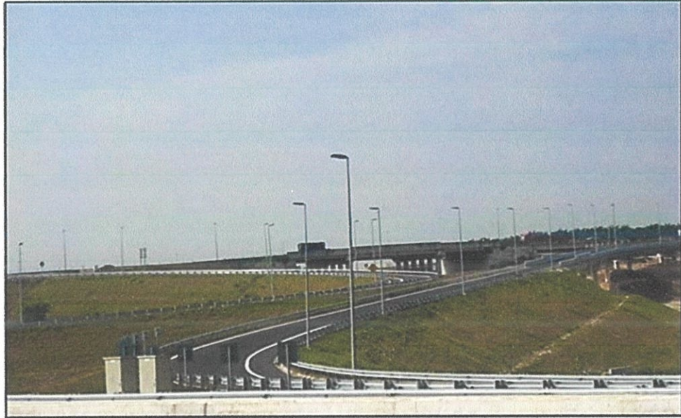
Figure 2.5: Kuala Lumpur – Kuala Selangor Expressway (KLSE).
