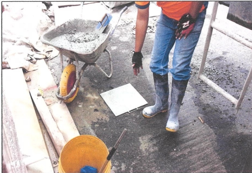
Photo 3.2: The base plate is put on the smooth surface.
