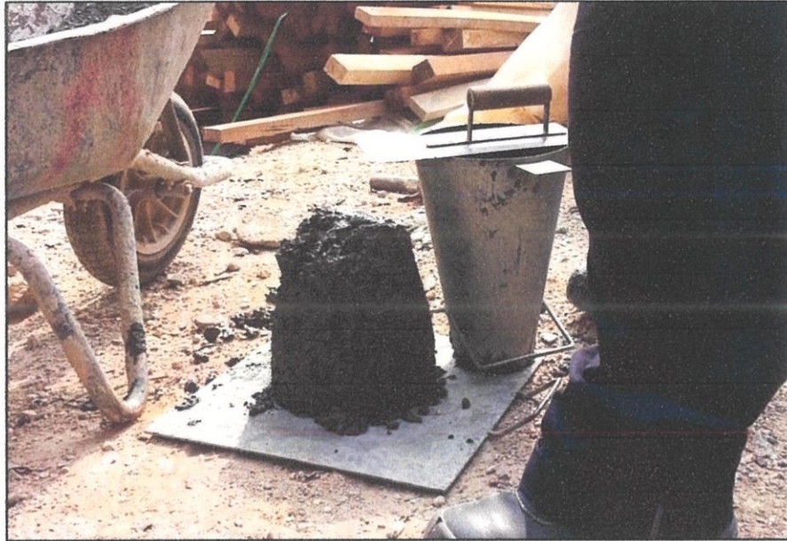
Photo 3.8: The frustum and scrapper is placed beside the concrete.
