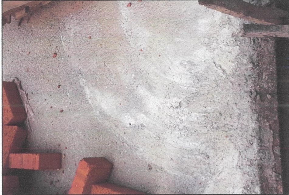
Photo 3.19: Efflorescence.
