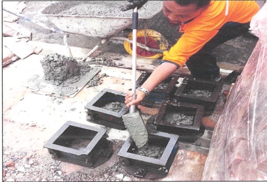
Photo 3.11: The mould is fill with concrete.
