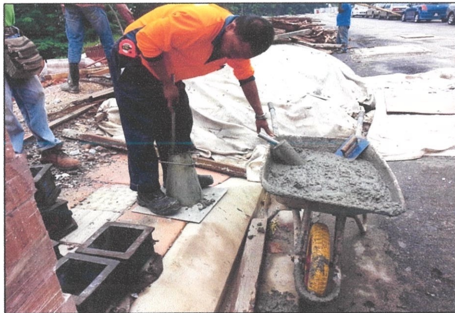
Photo 3.5: The concrete is temped for 25 times.
