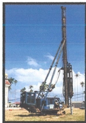
Photo 3.7: Example of Pile Driven Hammer Machine Used In the Case Study
