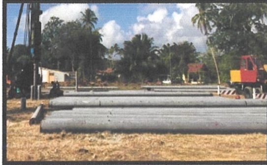
Photo 3.2: Spun Pile Used For This Case Study
