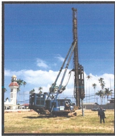
Photo 3.3: Driven Hammer Machine Started the Piling Work
