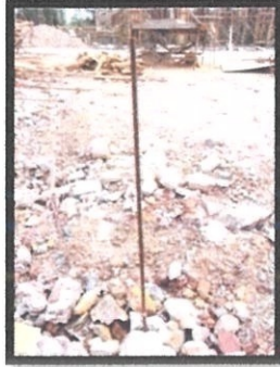
Photo 3.8: Example of Steel Rod Use in the Case Study
