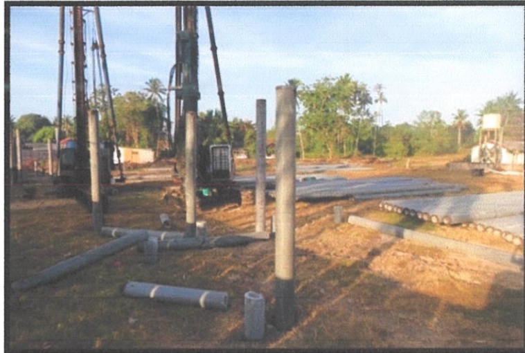
Photo 3.4: Driven Hammer Machine Continued the Piling Work
