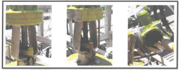
Figure 11 MOV 1D06 and MOV 1D07 broken and dislodged.
