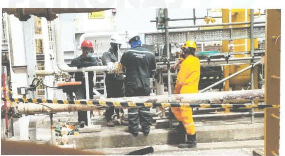
Figure 34 Contractors removing insulation on the pipeline.
