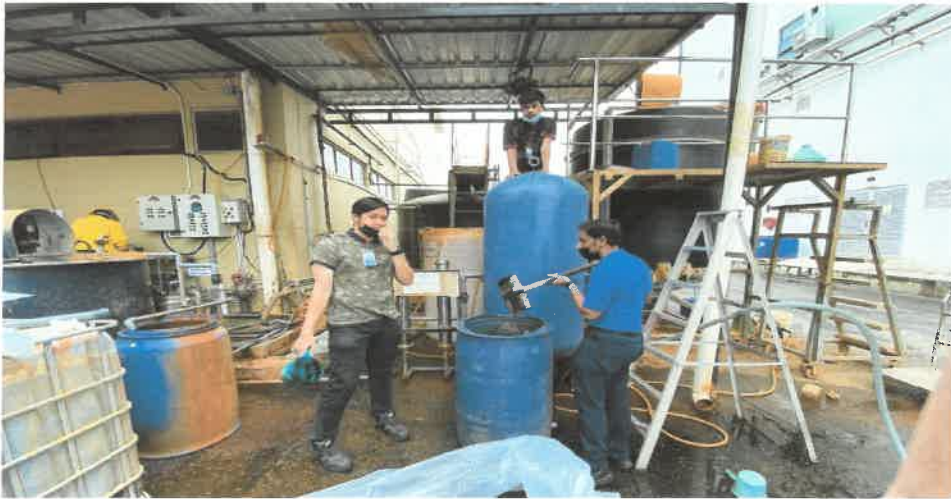
Figure 16 Activated carbon filter tank (blue)
