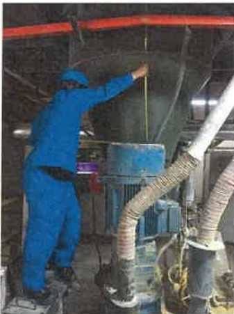
Figure 18: Measure the tank with supervisor.
