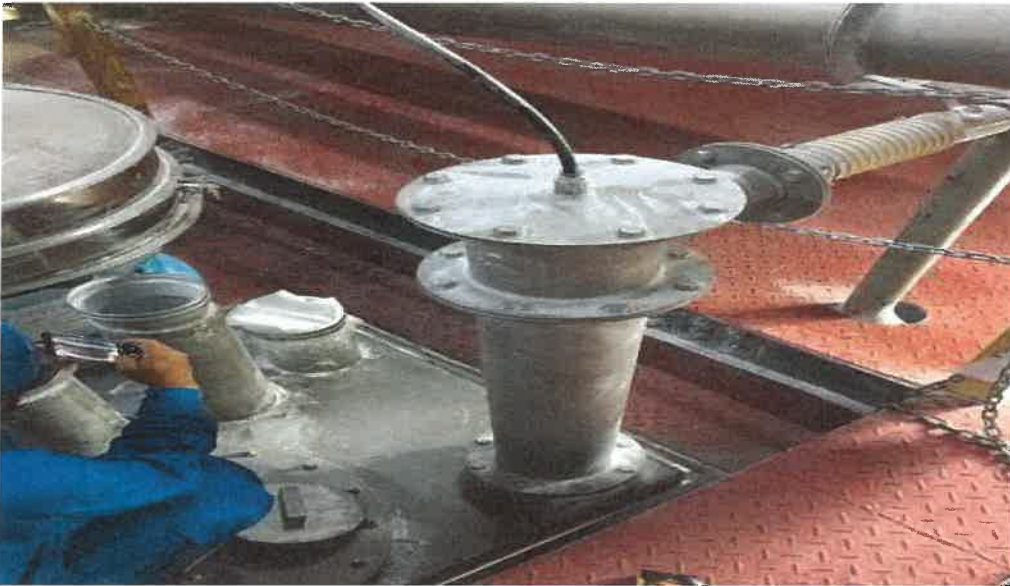
Figure 14 : Measure the hole with supervisor.
