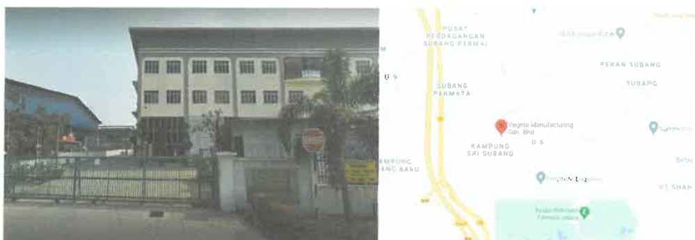
Figure 1: Front view and location of Vegeta Manufacturing Sdn Bhd.
