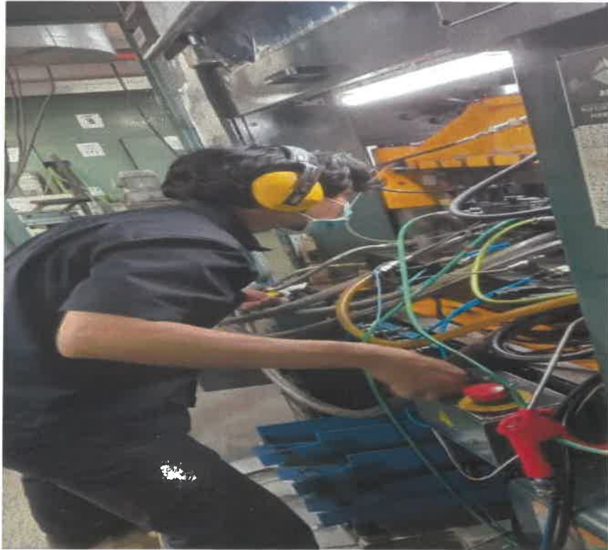
Figure 2.4.2 : Setting coil using inching method and position while setting coil in Dyson V10 press machine (DIE)
