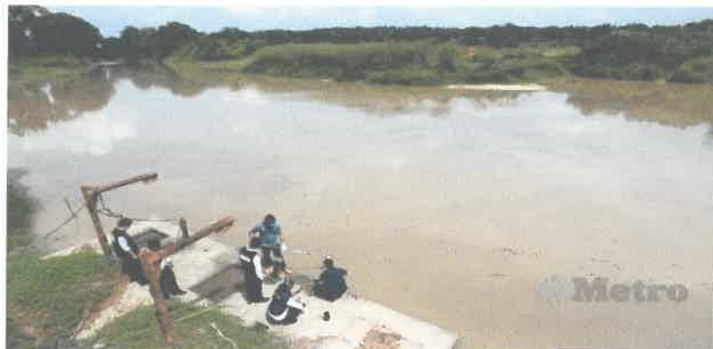
Figure 18 : Intake of Keratong Water Treatment Plant
