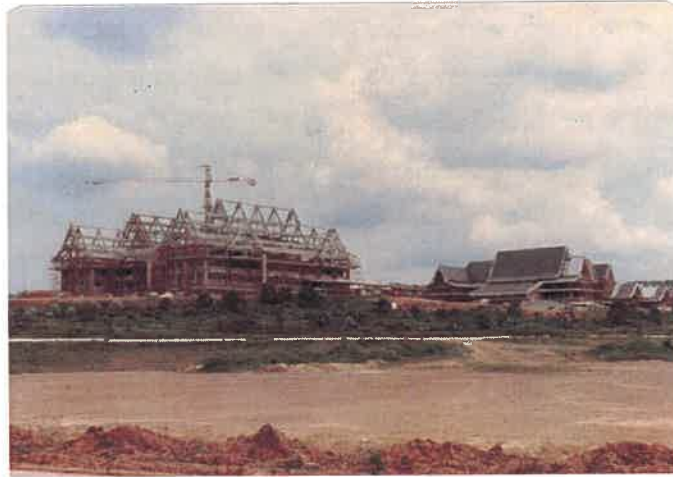
Figure 2.5: New Campus Construction at Skudai, Johor in 1985
