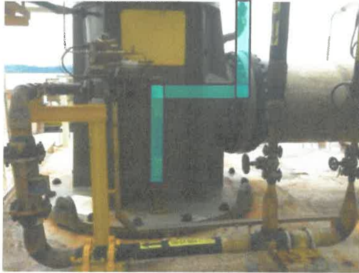
Figure 15: Piping system for Electrolyzer
