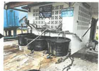
Alum, Soda, Polymer mixing tank
